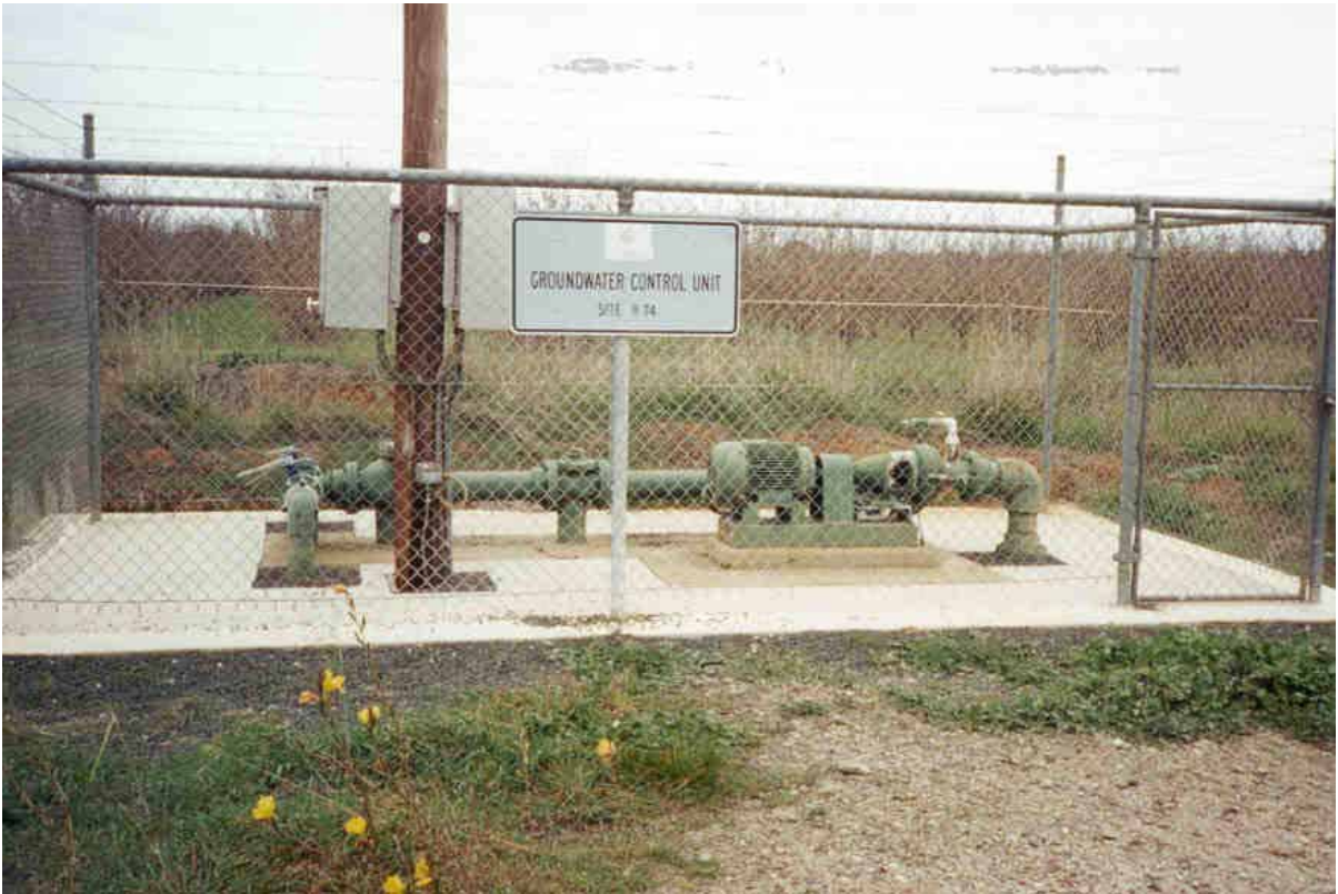
Pump for subsurface drainage by vertical drains (J.W. Hornbuckle)
