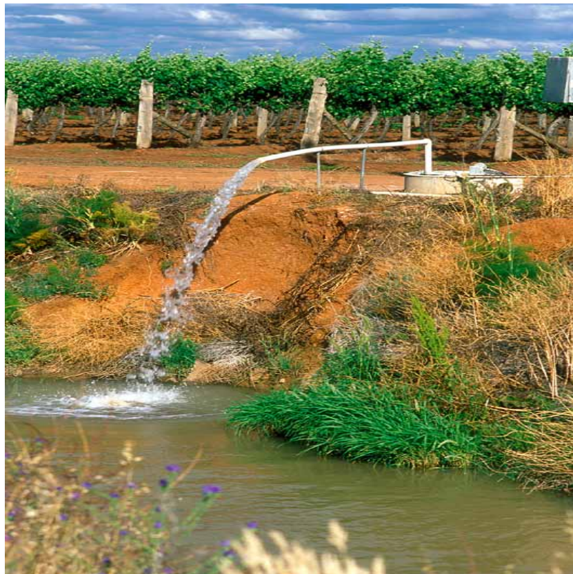
Subsurface drainage pump (pipe drains) discharging to surface drain in the MIA (E.W. Christen)
