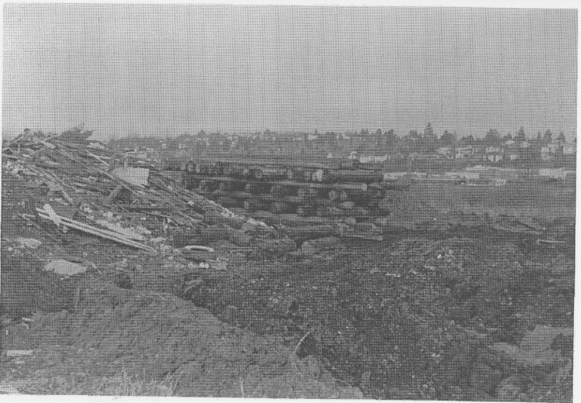
Figure 22: Picture of timber dikes in Montlake landfill January 1960
