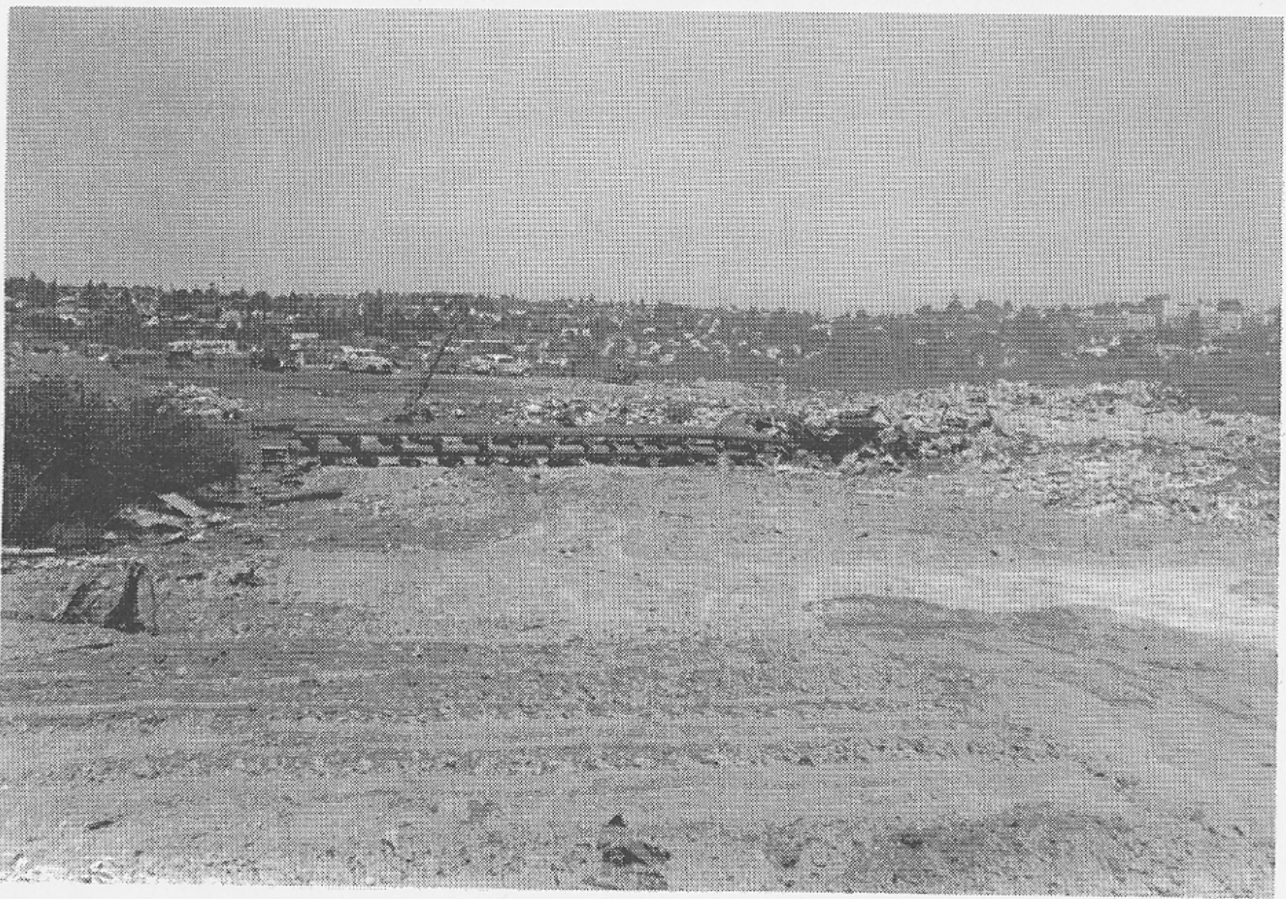
Figure 23: Picture of timber dikes in Montlake Landfill July 1961
