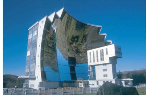
FIGURE 255 The last mirror of the solar furnace at Odeillo, in the French Pyrenees (© Gerhard Weinrebe)
