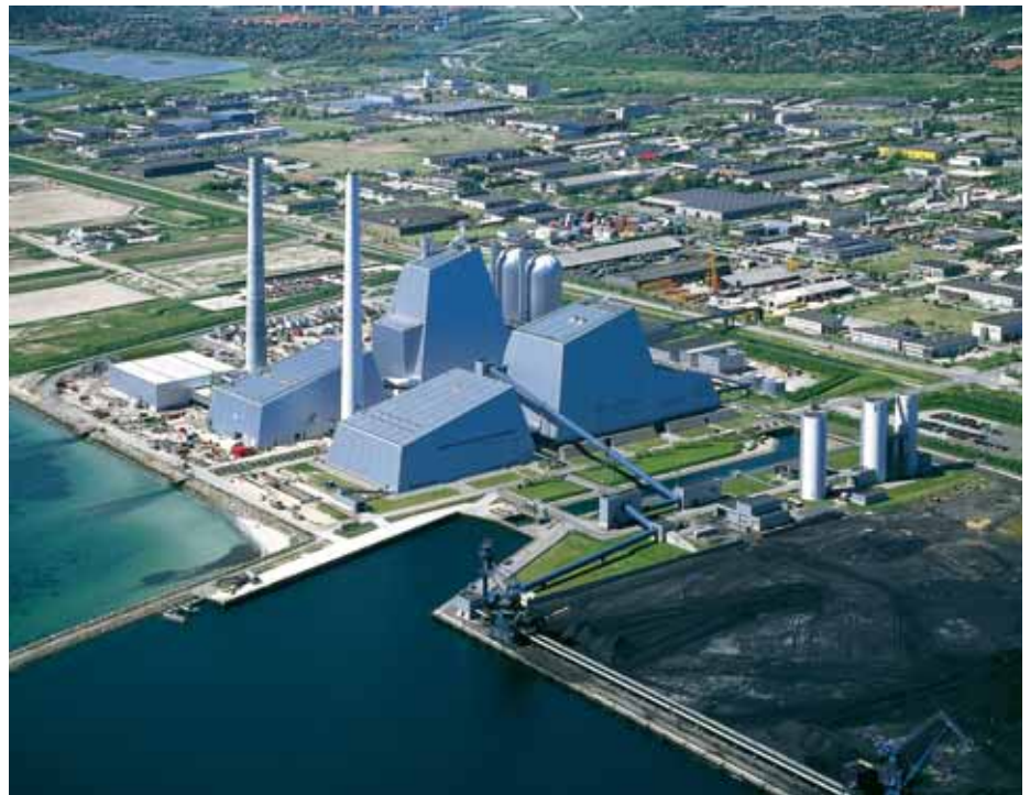
Avedøre CHP plant. From right to left: coal storage, unit 1, unit 2, and straw storage. Two heat accumulators behind AVV2. (Photo: Energi E2).
