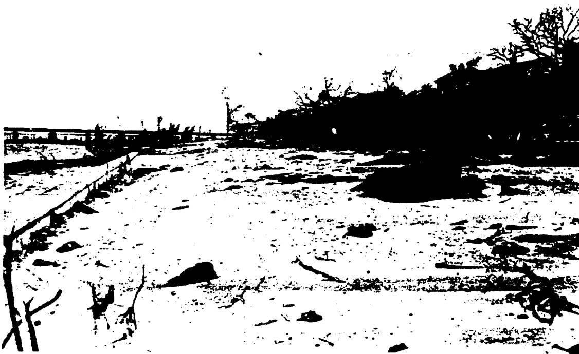
EROSION OF FRONT ROAD AT BAY ST. LOUIS L & N RAILROAD BRIDGE IN BACKGROUND
