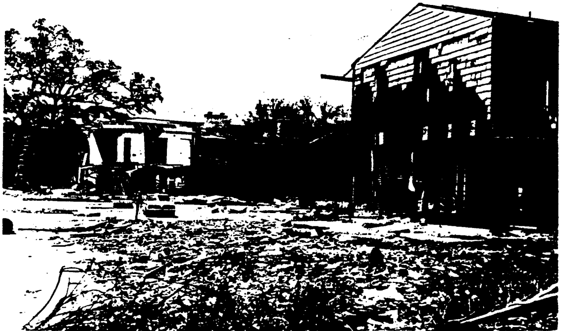
FIRST FLOOR OF THIS APARTMENT WASHED OUT, LEAVING THE FRAMING TO SUPPORT SECOND FLOOR
