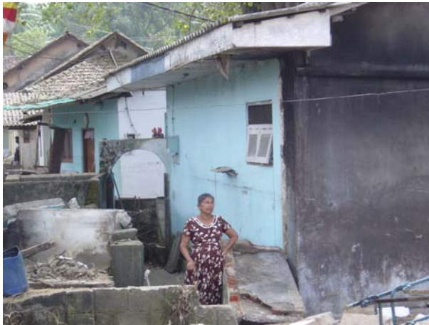
Photo 11 Barely damaged houses behind the Beruwala fishing harbour
