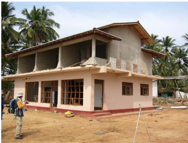
Photo 13 Barely damaged building made of concrete
