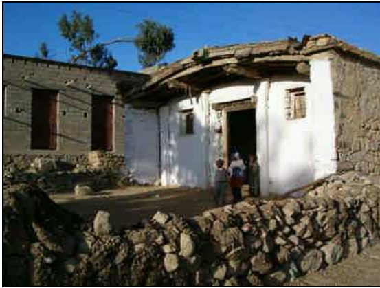
Figure 3-2: Front side of a hidmo in Emba Derho (photograph by L. Lätt, 2004)
