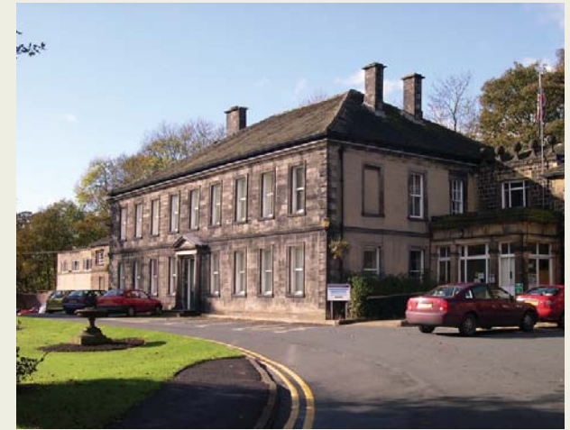
Bingley Town Hall
