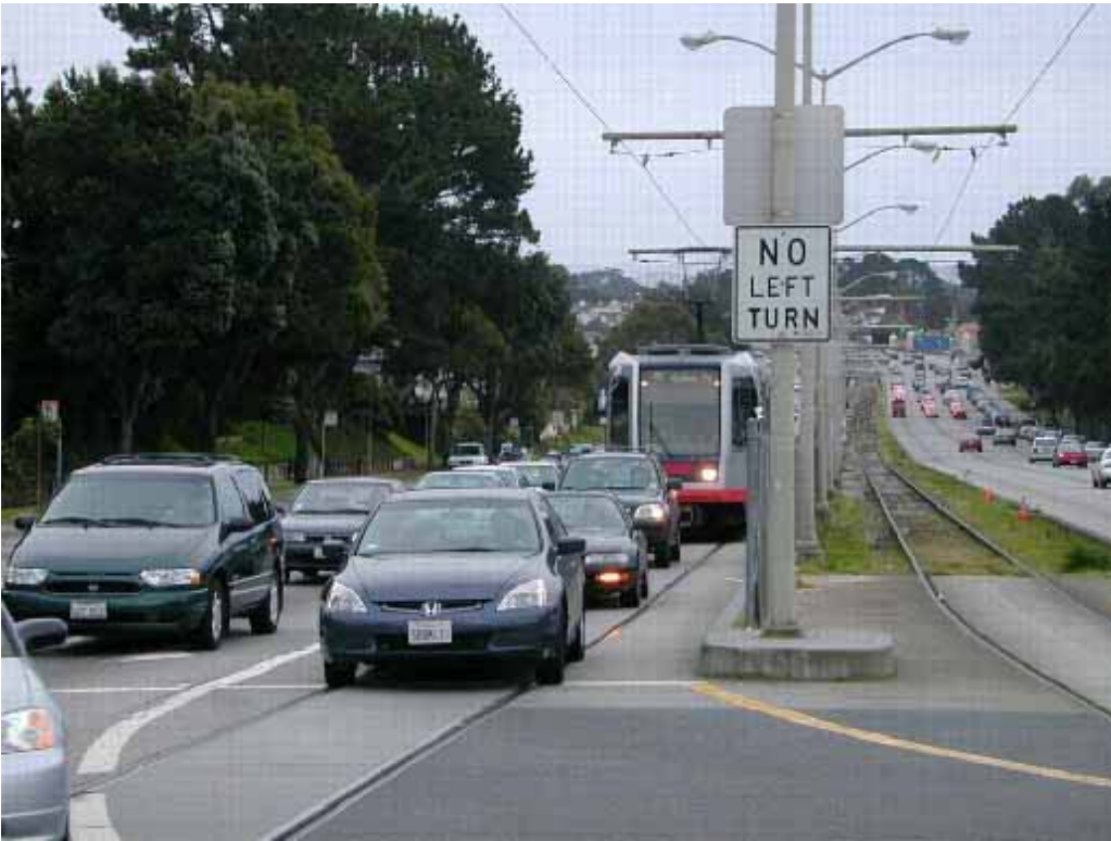
Figure 7. Left turn lanes, San Francisco Muni, with pavement around rail tracks to indicate shared rail and vehicle use. Track is not paved except for shared left turn lanes.
