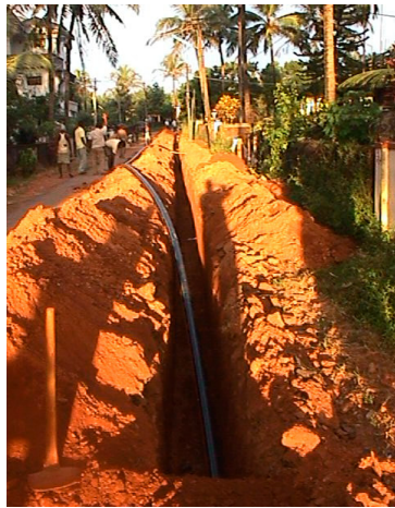
Udupi pipe installation in progress
