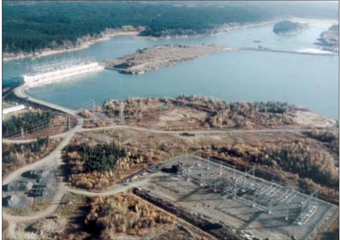
This aerial view of the Kelsey Generating Station shows the powerhouse (upper left) and the spillway (far upper right) a short distance away. The geography of the area did not lend itself well to having the spillway built "run-of-river" — that is, built adjacent to the powerhouse.
