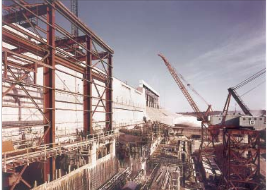
During part of Kettle's construction — between 1966 and 1973 — the water flow of the Nelson River was diverted through the spillway while the powerhouse was being built on the cofferdam, a dry area created in the middle of the river.
