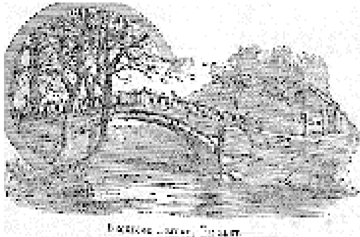
Beckfoot Bridge, Bingley.
