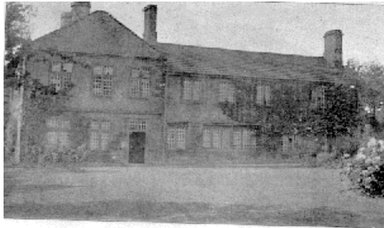
THE OLD VICARAGE, BINGLEY.
