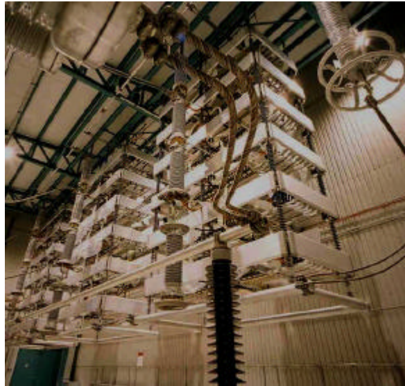
LTT quadruple valves assembled on site
