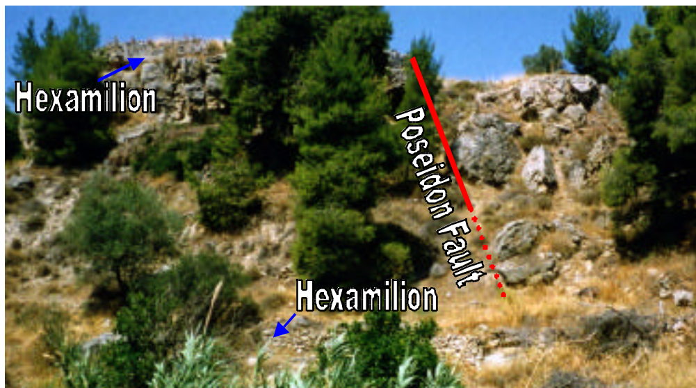
Fig. 2. The Poseidon fault is crossed in several locations by the Hexamilion, and underlies much of the central extent of this ancient fortification. Here we see the offset in the surface caused by the fault.
