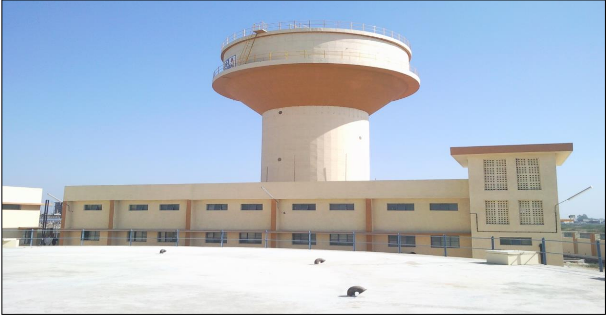
ESR-GSR WORK AT BAPOD UNDER VAJPAL NAGAR VIKAS YOJANA
