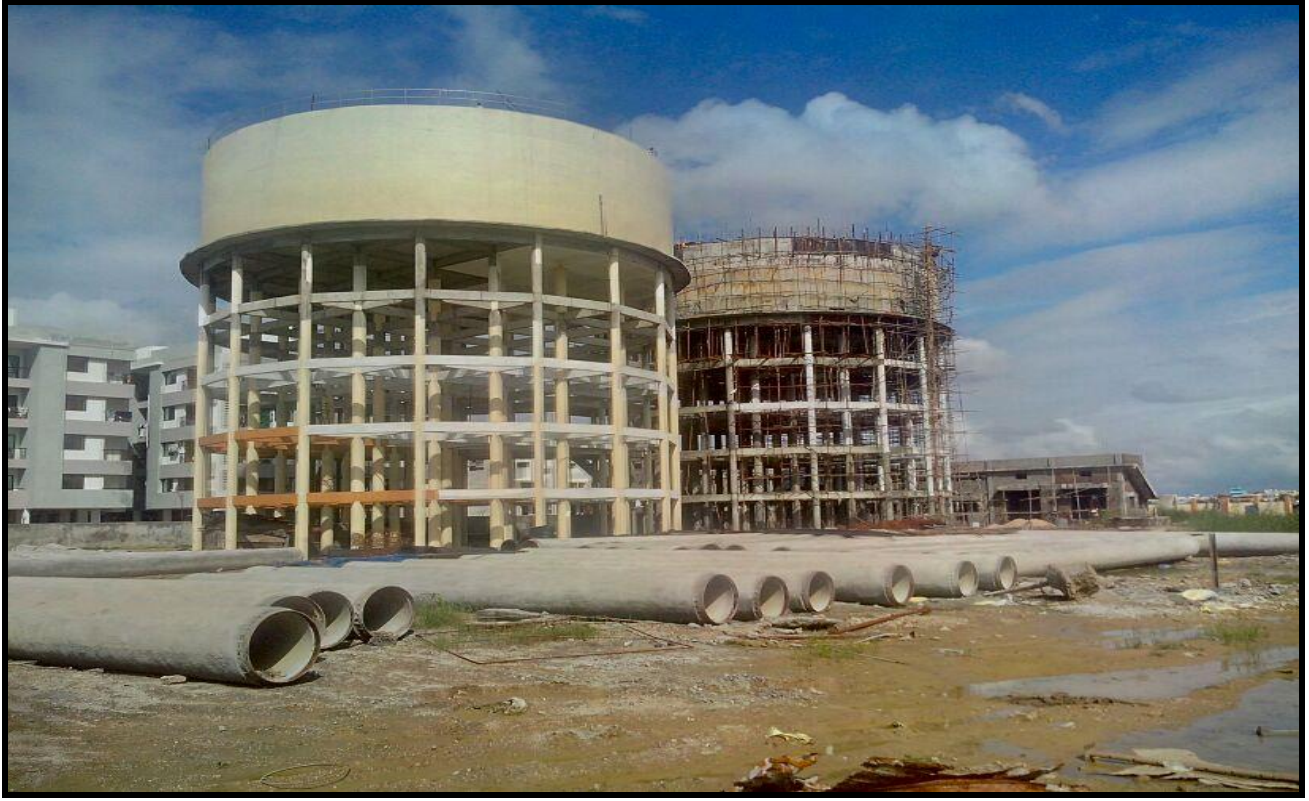
ESR-GSR WORK AT SAYAJIPURA UNDER 24X7 DPR(JnNURM)
