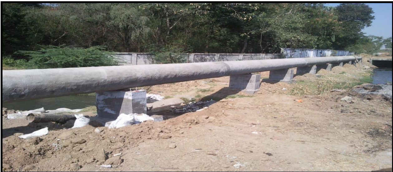
DI PIPELINE WORK AT JAMBUVA
