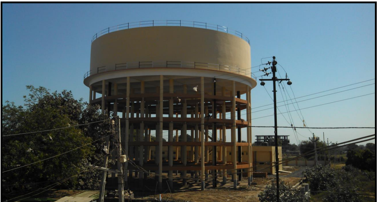
ESR-GSR WORK AT CHHANI UNDER 24X7 DPR(JnNURM)
