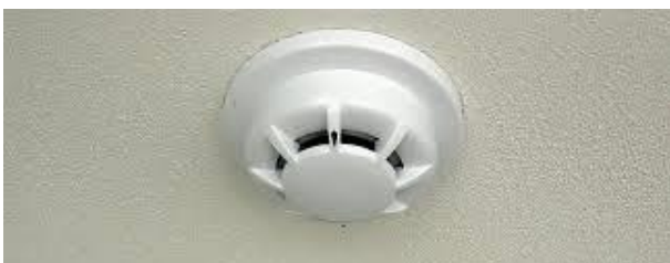
Figure 18: Smoke Detector
