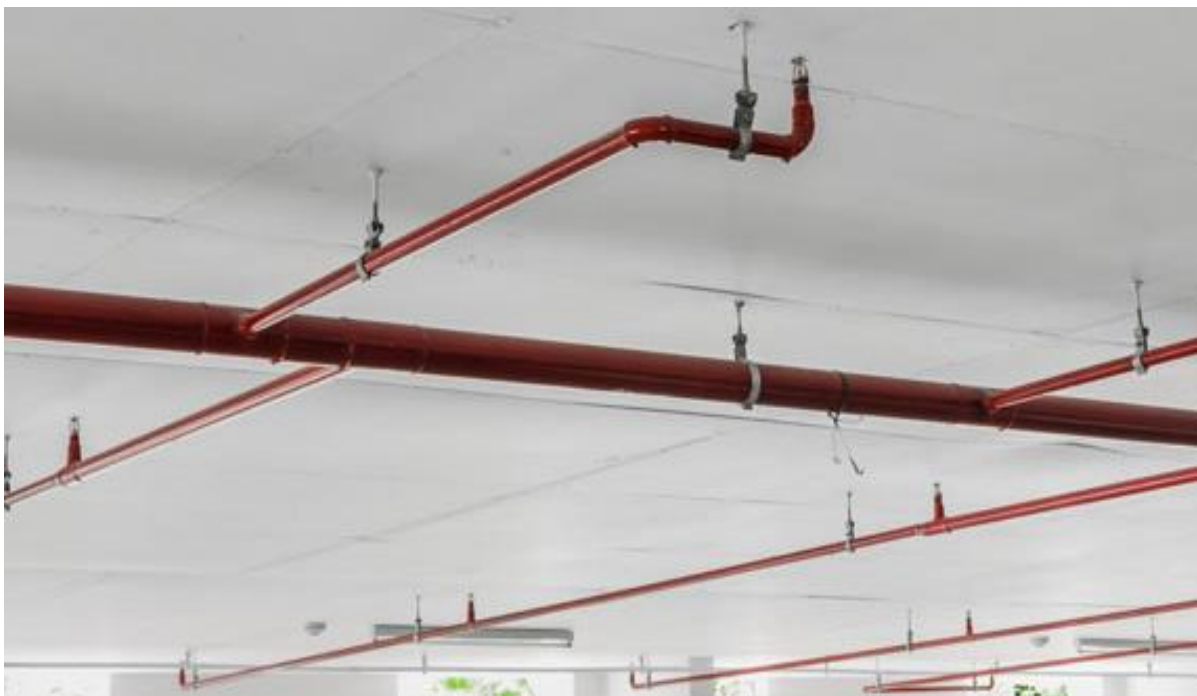
Figure 25: Automatic Sprinkler System
