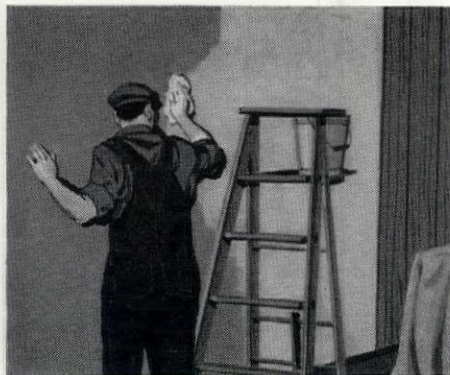
Air cleaner supervision
