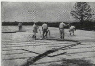
Pumping and screeding Zonolite concrete.
