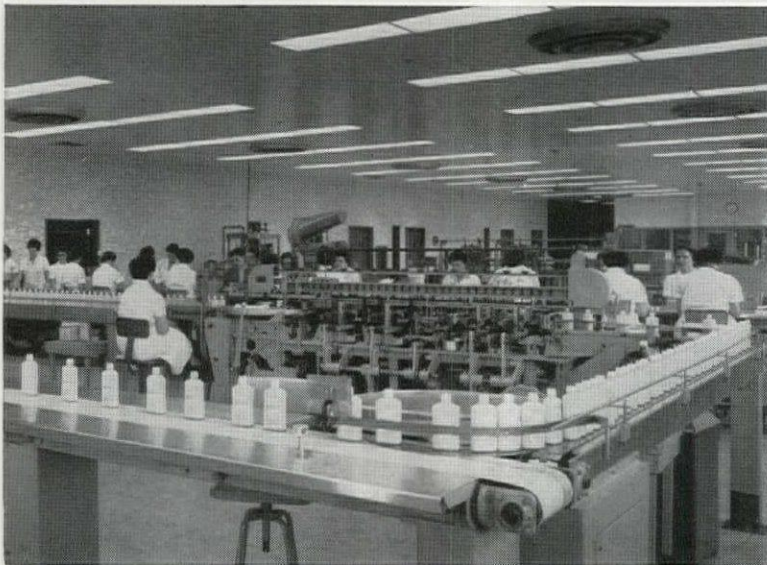
Listerine, Richard Hudnut, Du Barry and other famous name products are made here. Johnson Controls keep this air conditioned packaging area as comfortable as an executive office.
