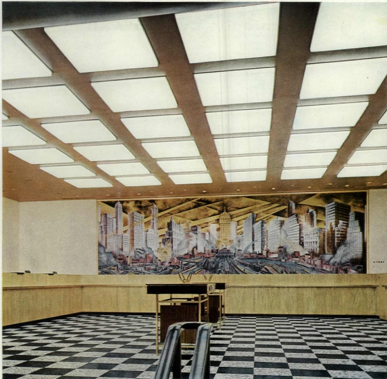
4'-square PLEXIGLAS diffusers at Park Avenue office of a large New York City bank
