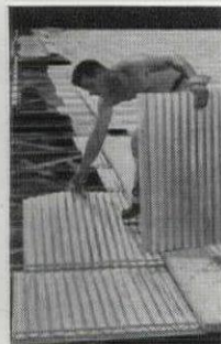
Placing corrugated decking on trussed tees.
