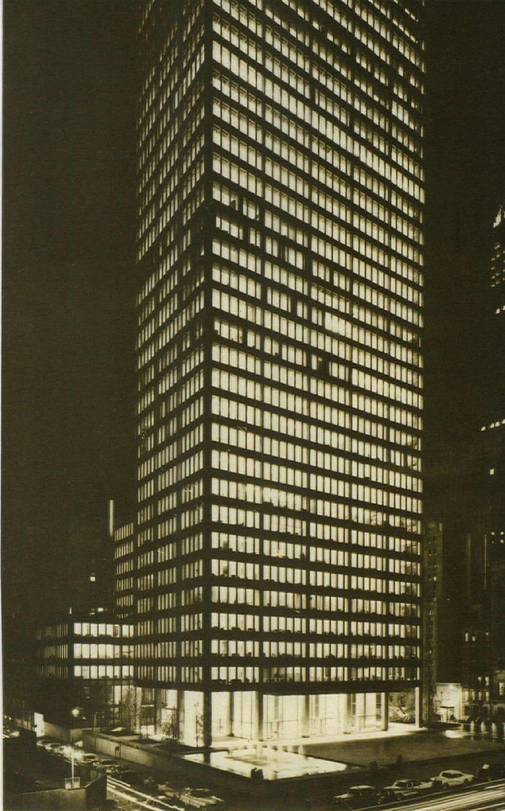
Photos: Ezra Stoller
