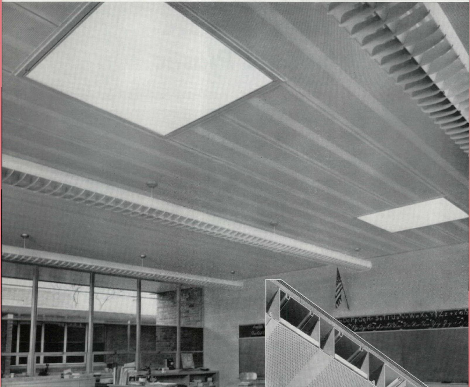
Classroom in Roosevelt School, Livonia, Michigan. One of Five new Schools in Livonia constructed with combined Roof-Ceilings in which the Mahon Long Span M-Deck provides the Roof Structure and the Acoustical Ceiling in one economical unit. Architects: Jahr-Anderson-Machida Associates, Inc. General Contractors: Birchard & Roberts.
