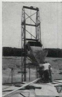
Hoisting mixed Zonolite concrete to concrete pump on roof deck.
