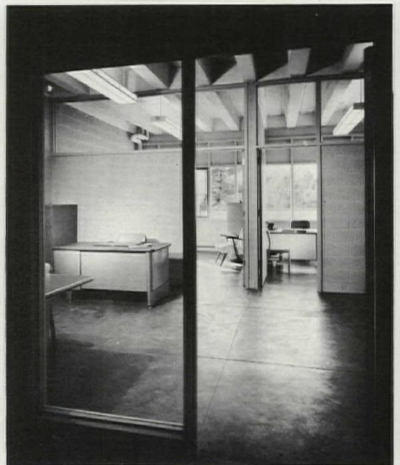
Lightweight block is used for partitions in such rooms as the card room on the main floor (above) or offices on the lower floor (right). Ceilings, in the main, are corrugated, perforated aluminum supporting an absorptive, acoustical blanket.
