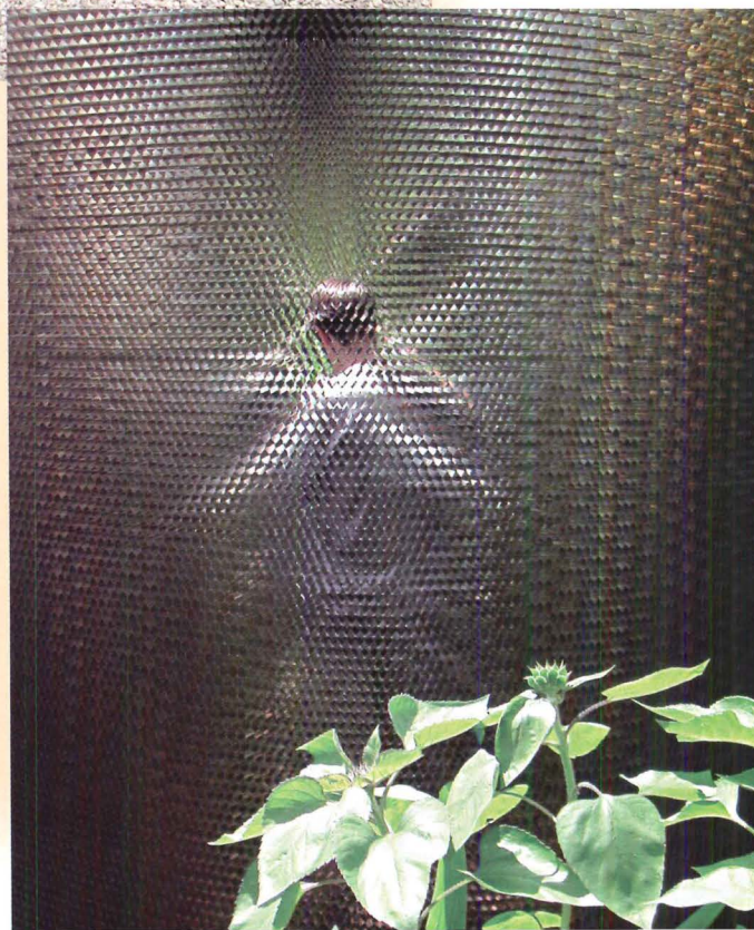
Sharon McHugh and John Nastasi Architects built the Cornel West Pavilion in 2004 with Nastasi's graduate students at Stevens. This temporary, self-supporting structure on the campus of Princeton University is made from a honeycomb metal mesh used in the aerospace industry. Its geometry was derived from a digital study of the material's structural properties.
