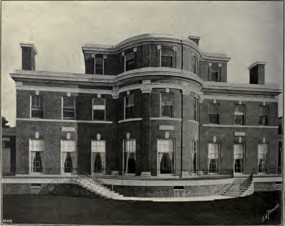
THE CENTRAL WING—MR. T. JEFFERSON COOLIDGE'S HOUSE.
