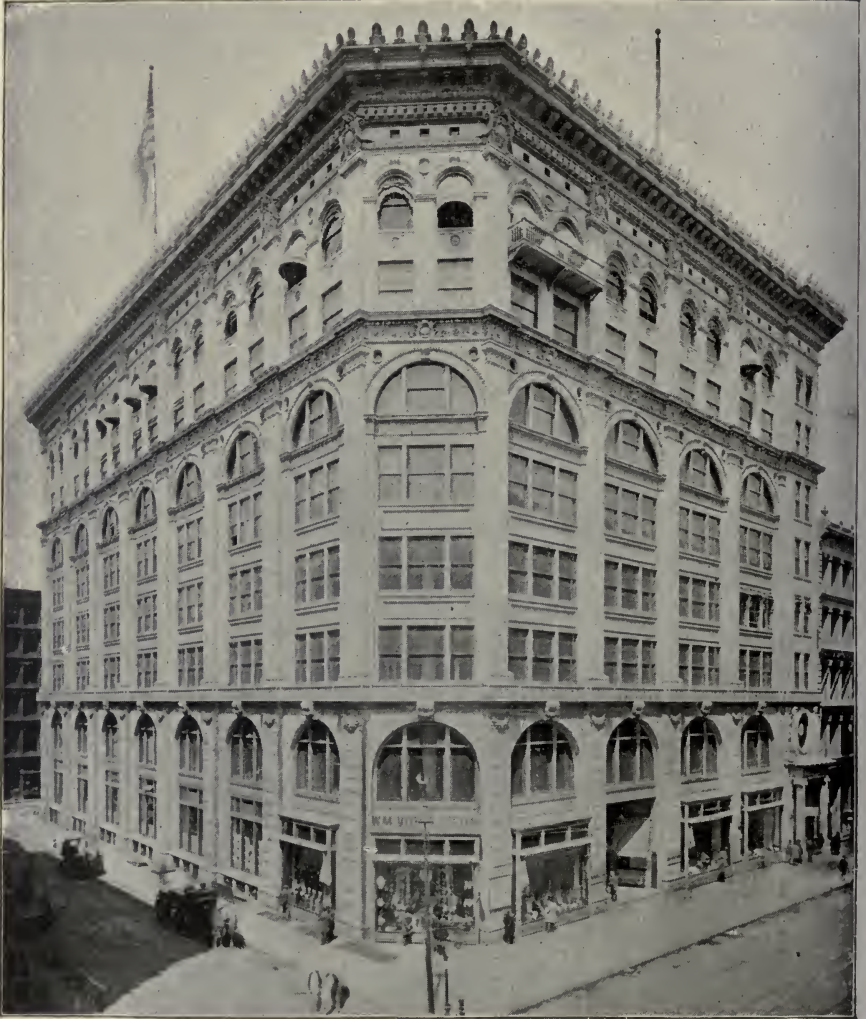
THE CABLE BUILDING.
