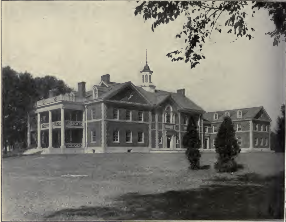
THE WOMEN'S BUILDING—UNIVERSITY OF ILLINOIS.
