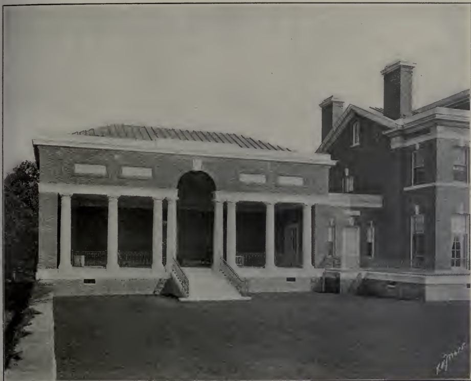
THE LOGGIA—MR. T. JEFFERSON COOLIDGE'S HOUSE.
