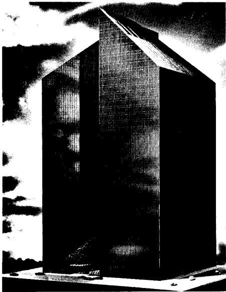
Pennzoil Place Houston, Texas Photo by Ezra Stoller
