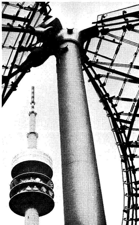
These details of the big roof, just before completion, show it suspended over the swimming stadium (opposite above); swooping down over the entrance area (opposite below and near right); and hung from towering, metallic tent spikes over the Olympic Stadium (above) where floodlights, each a meter in diameter, are attached to the chief bridge cable (far right).
