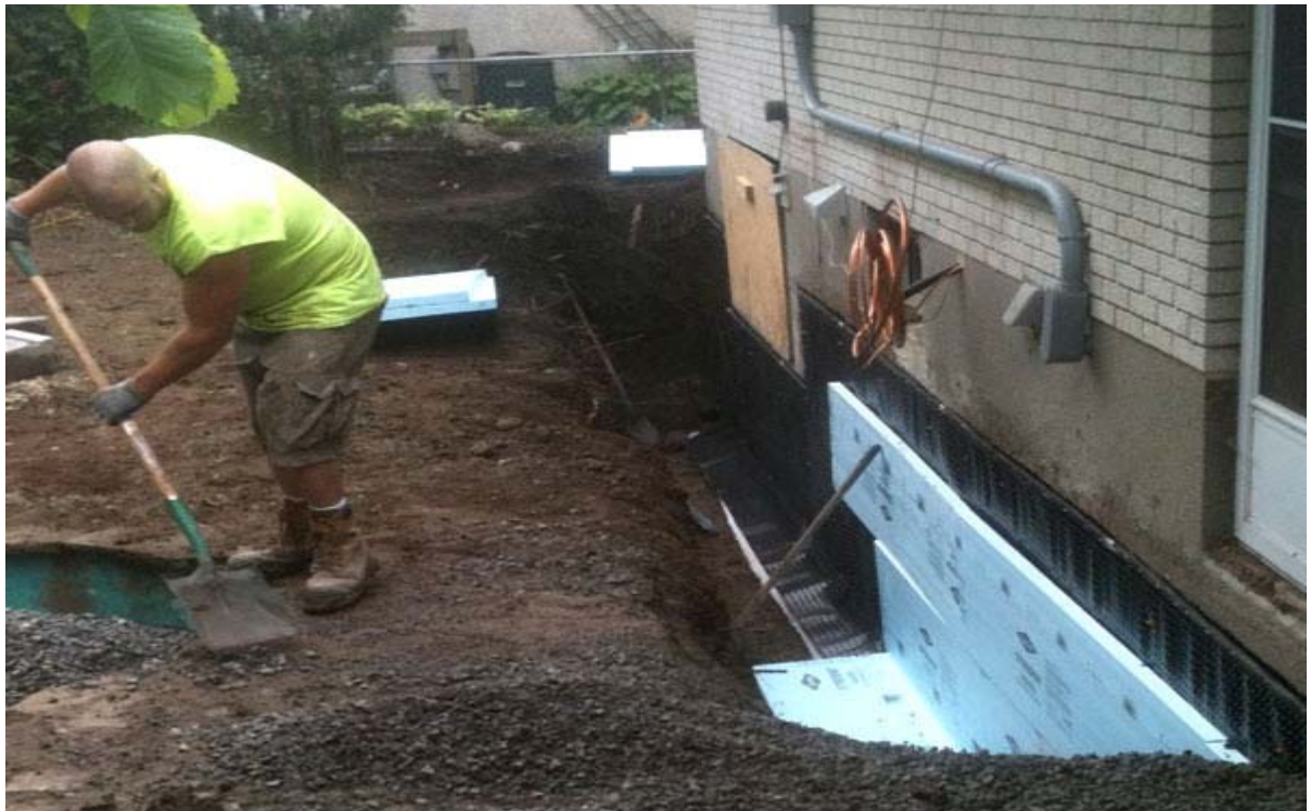
Fig. (4.2) Waterproofing of foundation
