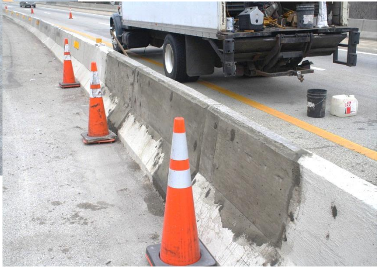
Median Wall Repair
