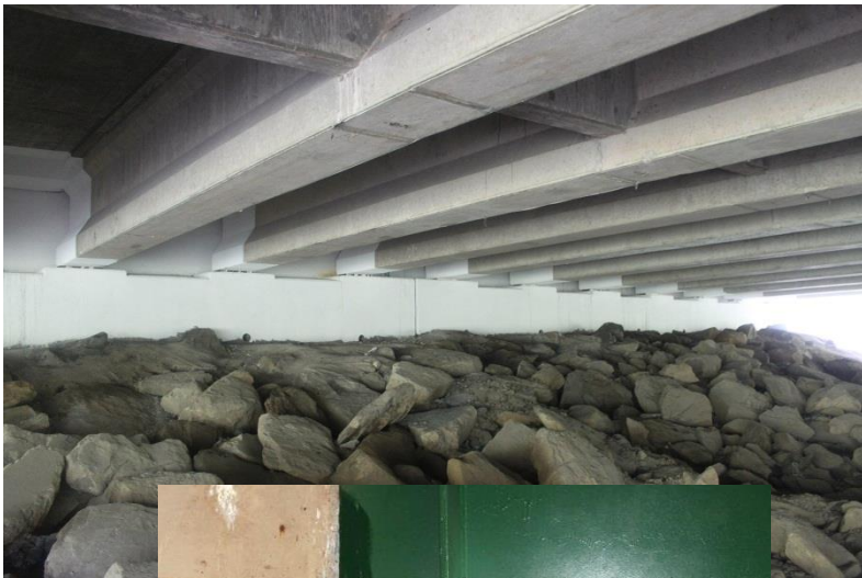
Abutment Cleaning & Painting
