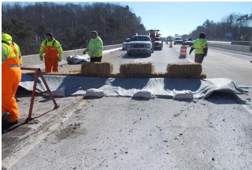
Deck Joint Repairs
