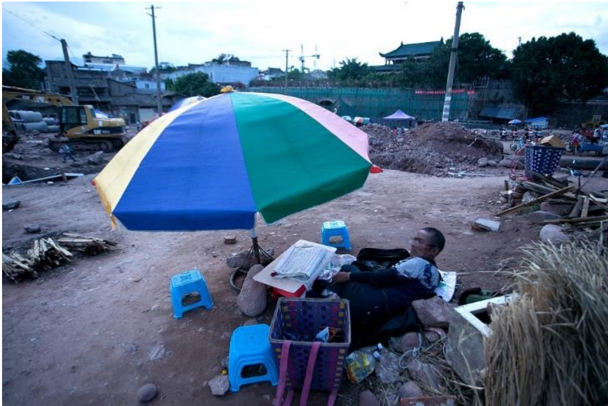
Figure 7: A process of destruction of the Shimazi's original location with ritualist facing the excavator (late summer 2016)
