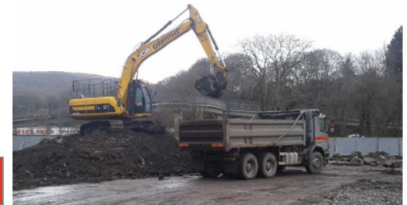
Right: Arisings being saved from land fill to be put to good use elsewhere
