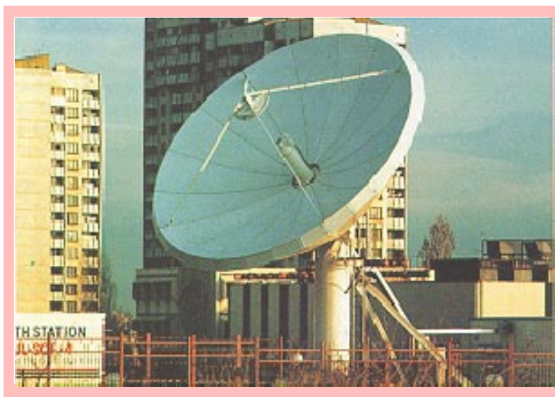
Figure 2 The earth station at Sofia (Bulgaria) where, fortunately, the urban development was behind the antenna.
