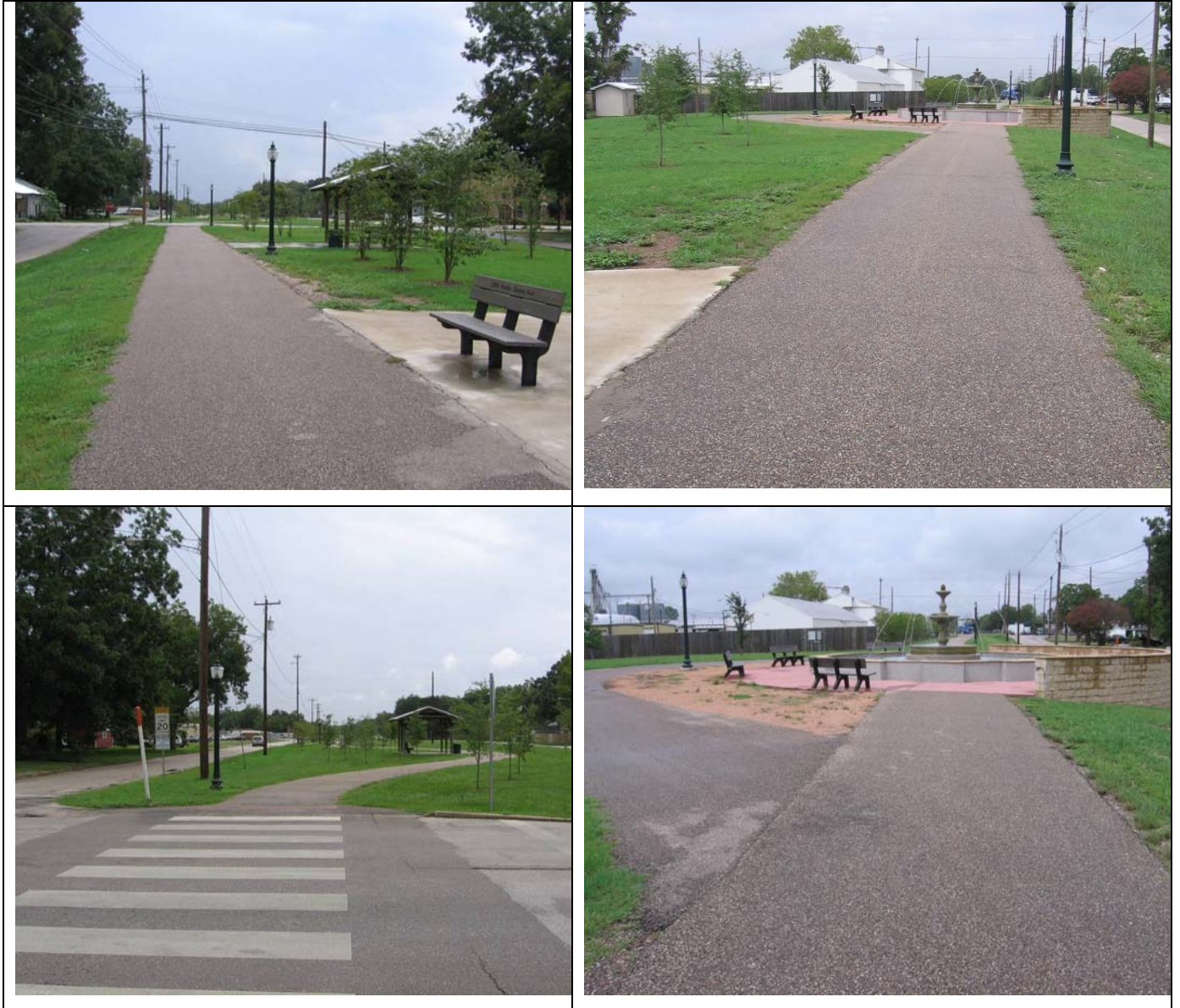
Figure 20. Wharton, Texas, Linear Paved Trail on Former GCSF Right-of-Way.
