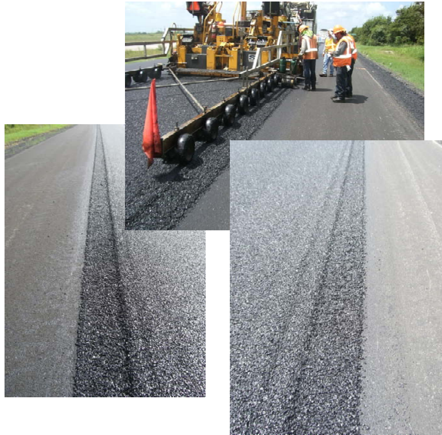
Figure 7. Notched Wedge Joint Construction in PFC.
