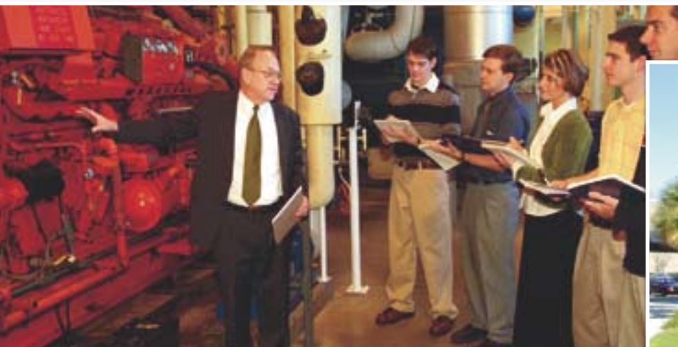
Dr. McLaughlin shows students an engine in the Cogeneration Building.
