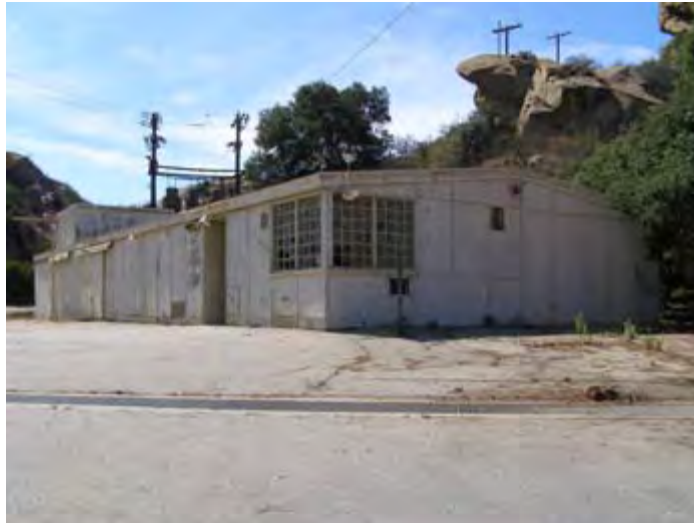
Photo 4.62. Delta Pre-Test Building, camera facing southeast. (Source: Archaeological Consultants, Inc., 2007.)
