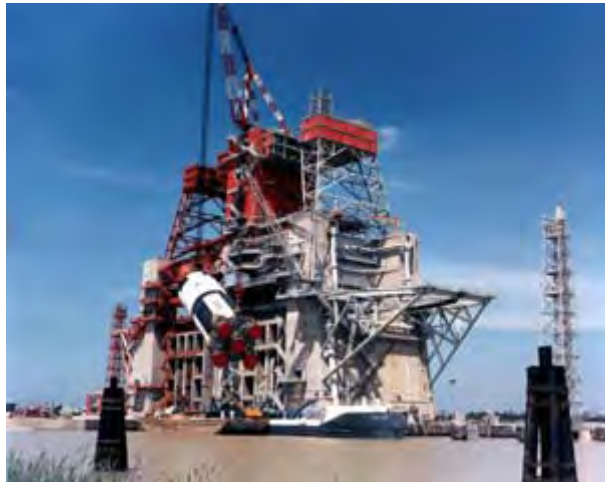
Photo 3.24. Installation of S-IC booster on test stand at the Mississippi Test Facility (today's Stennis Space Center), 1967. Five F-1 engines powered the S-IC, the first stage of the Saturn V.
