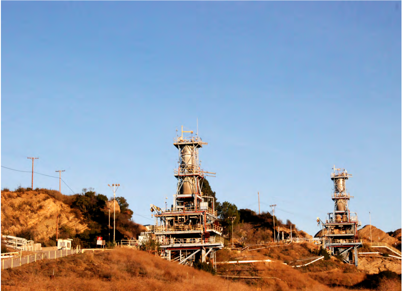
Photo 4.15. Alfa Test Stands II and III (Source: MSFC Historic Preservation Archives)
