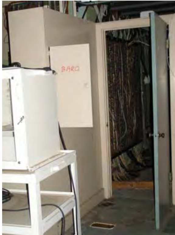
Photo 4.24. Bravo Terminal House, interior, camera facing east. (Source: Archaeological Consultants, Inc., 2007.)
