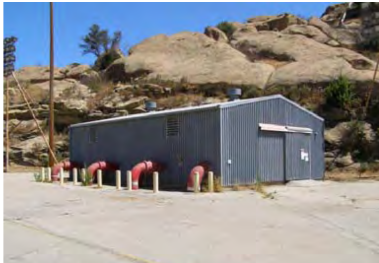
Photo 4.47. Pump House, camera facing east. (Source: Archaeological Consultants, Inc., 2007.)
