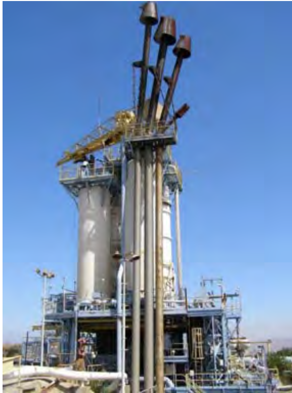
Photo 4.33. Bravo II Test Stand, west elevation. (Source: Archaeological Consultants, Inc., 2007.)
