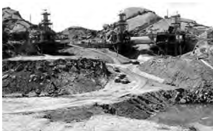
Photo 3.20. Delta site at AFP 57 (NASA Area II), 21 May 1957. Delta I, II, and III test stands, pre-test building, and fuel infrastructure (center), with wooden staircase to pill box (center to background right).
