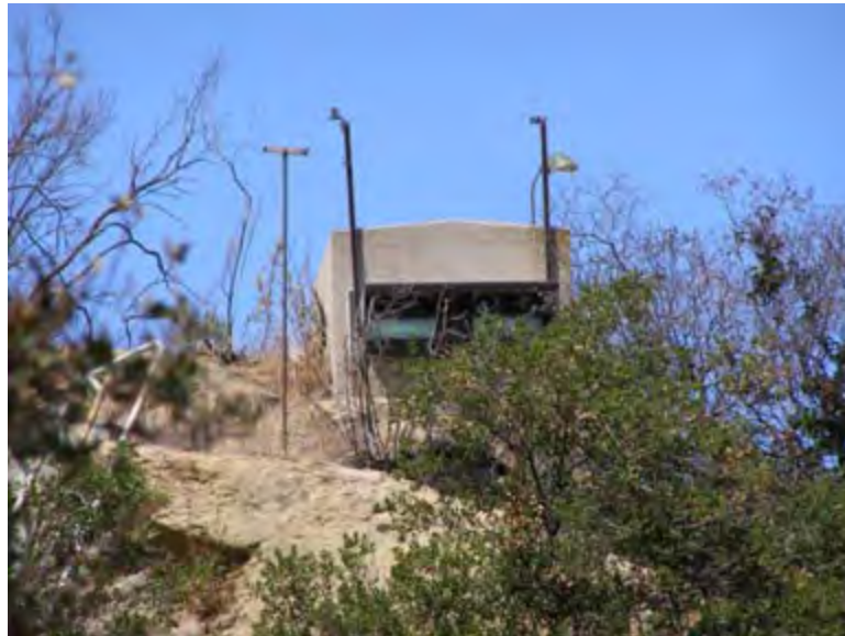
Photo 4.23. Bravo Pill Box, camera facing south. (Source: Archaeological Consultants, Inc., 2007.)
