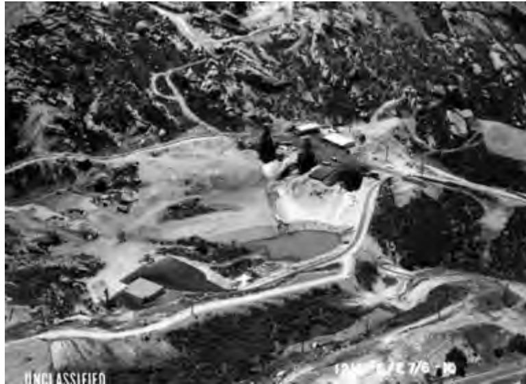
Photo 4.21. Bravo Test Stand construction, June 1956, camera facing northwest. (Source: Boeing Company/Santa Susana Field Laboratory; Photo #694.)
