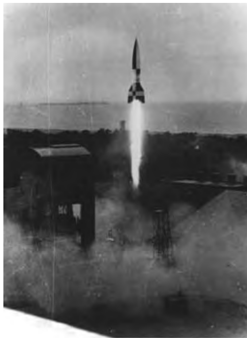
Photo 3.7. Launch of a V-2 at Peenemünde, Germany, 1 January 1942. Test Stand VII consisted of a reinforced concrete launch pad with blast containment walls and a moveable gantry. (Source: History Office, Marshall Space Flight Center.)
