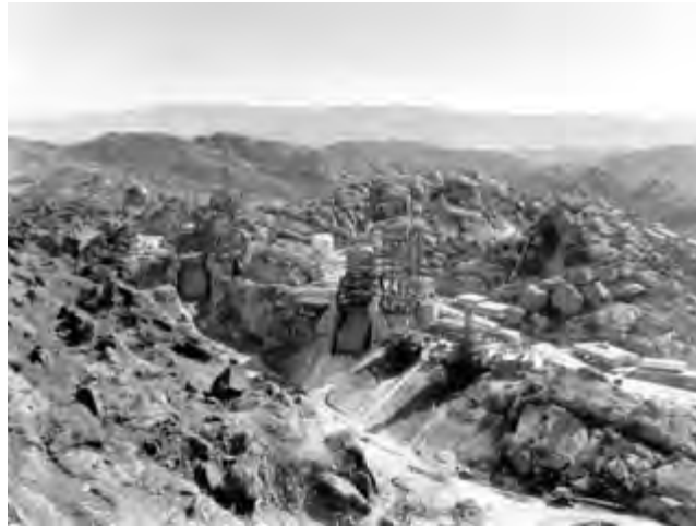
Photo 3.23. Coca site at AFP 57 (NASA Area II), 27 January 1964. Left to right: Coca IV, I (rebuilt), II (base only), and III. Lower pre-test building (foreground right), wooden staircase to 1950s pill box (center right), 1960s pill box (background center), and GH2 recovery system (“eight ball”) (background center left).
