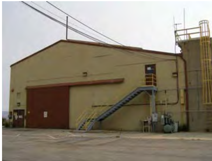
Photo 4.64. Components Test Laboratory (2206), camera facing northeast. (Source: Archaeological Consultants, Inc., 2007.)
