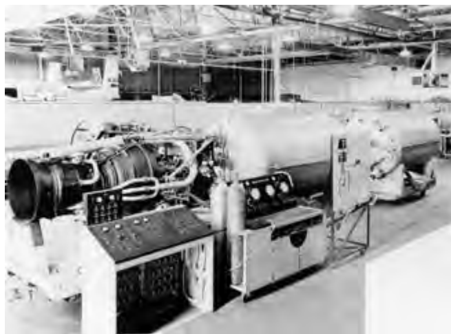
Photo 3.9. MX-770 Navaho Phase 2 engine with propellant tanks, at the North American Aviation plant in Downey, 13 September 1949.
