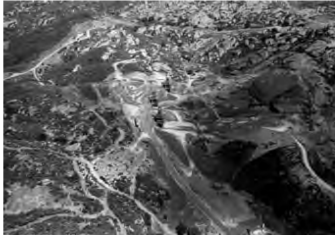
Photo 3.14. Alfa site at AFP 57 (NASA Area II), 3 June 1958. Pre-test building, Alfa I, II, and III test stands, underground blockhouse facing the spillway ravine (foreground right), pill box (center right), 24-inch aboveground pipeline to water storage tanks (background to upper right corner), and fuel infrastructure.
