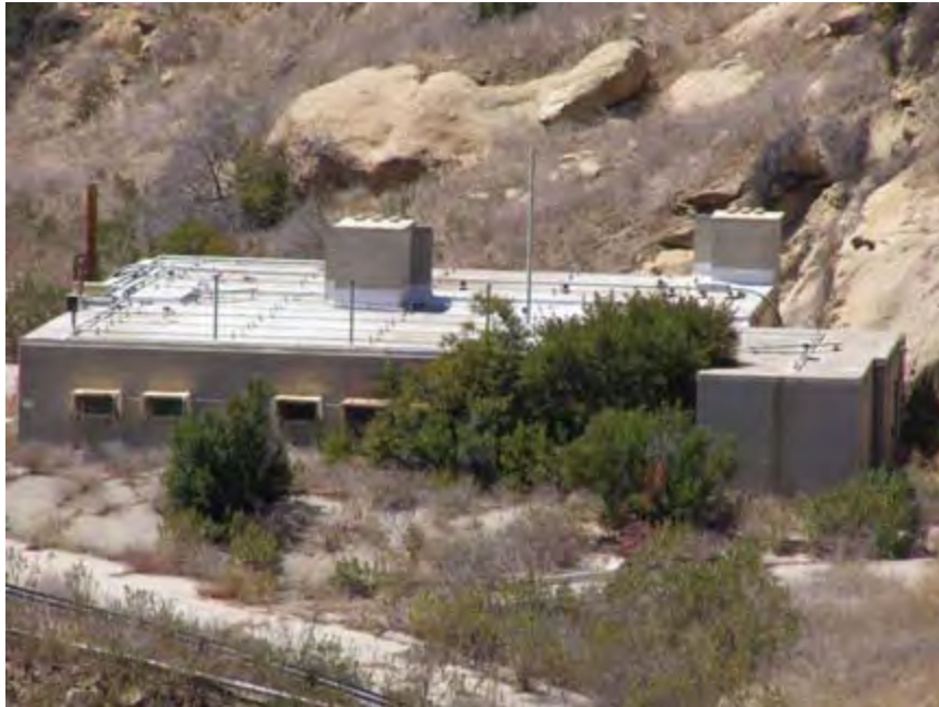
Photo 4.58. Coca Control House, east elevation. (Source: Archaeological Consultants, Inc., 2007.)
