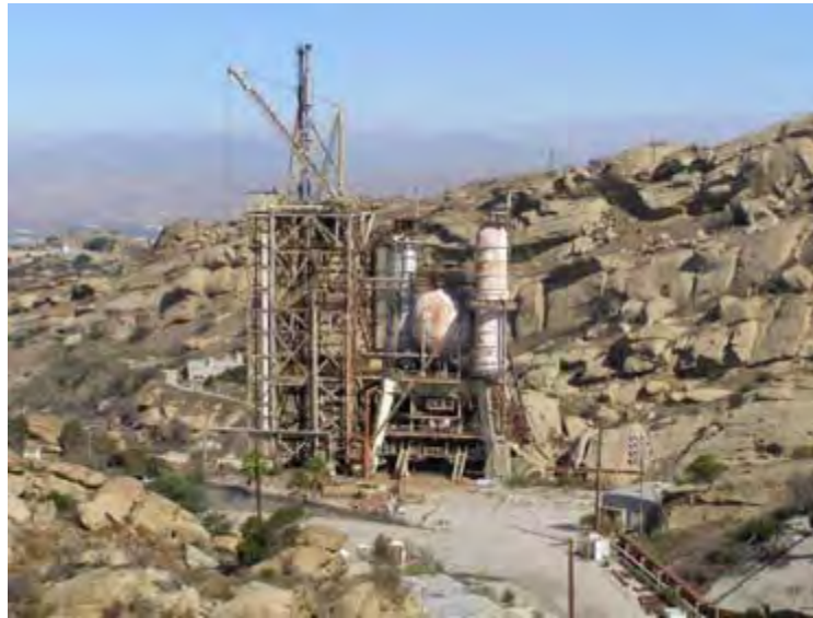
Photo 4.50. Coca I Test Stand, south elevation. (Source: Archaeological Consultants, Inc., 2007.)
