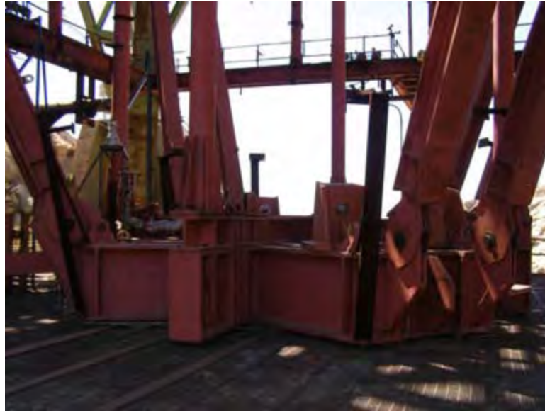
Photo 4.57. Coca IV Test Stand, working level, camera facing northwest. (Source: Archaeological Consultants, Inc., 2007.)
