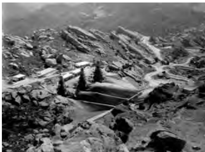
Photo 3.19. Coca site at AFP 57 (NASA Area II), 3 June 1958. Showing flame trenches cut through existing rock. Pre-test building, Coca I, II, and III test stands, and fuel infrastructure. Blockhouse not visible.
