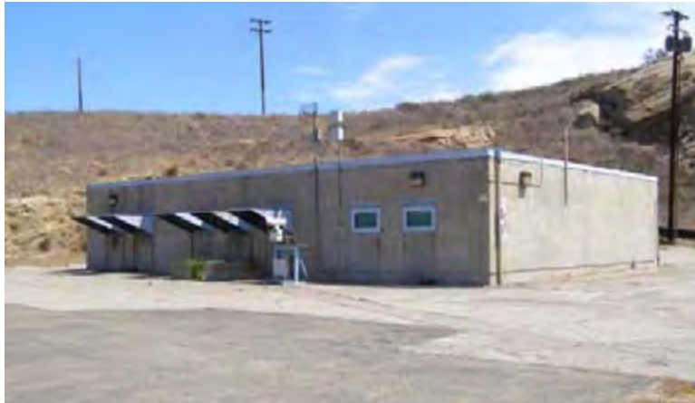
Photo 4.36. Bravo Control House, west and south elevations. (Source: Archaeological Consultants, Inc., 2007.)
