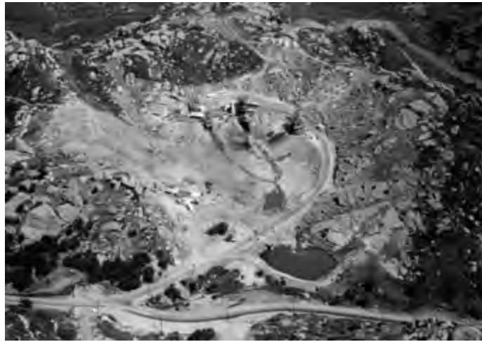
Photo 3.12. Aerial view of the Bowl Area at Santa Susana (Boeing Area I), 3 June 1958. Preparation stand, VTS I, II, and III, flame trenches and spillway, conservation dam (foreground), blockhouse (center), four water tanks (background), and fuel storage infrastructure.
