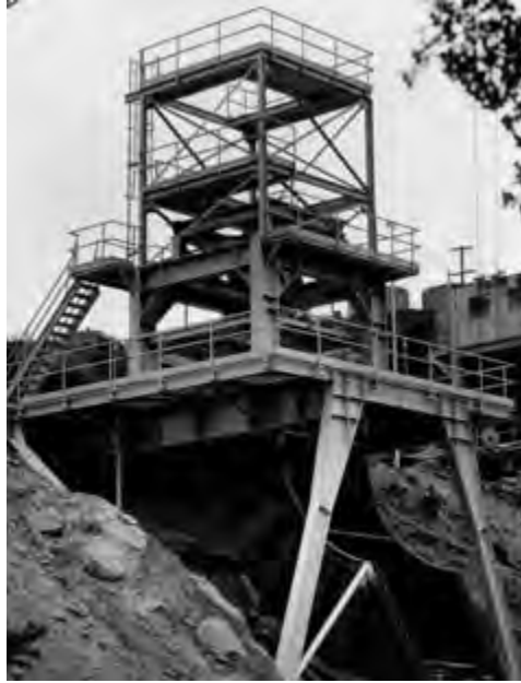
Photo 3.13. Canyon Area test stand at Santa Susana (Boeing Area I), 15 May 1953. (Source: Boeing, Rocketdyne Historic Photograph Collection, SSFL.)
