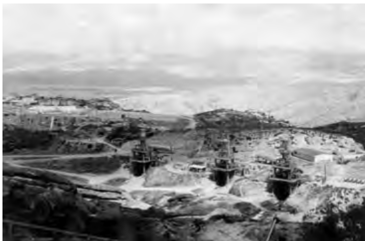
Photo 3.15. Alfa I, II, and III test stands (NASA Area II), with flame trenches emptying into the spillway ravine, 2 May 1959. CTS II (turbopump test facility) and edge of Service Area (both background left) and 24-inch water pipeline (foreground). (Source: Boeing, Rocketdyne Historic Photograph Collection, SSFL.)
