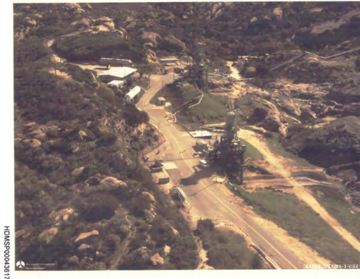
Photo 4.1. Alfa Area showing Test Stand No. I (Building 2727) in the foreground, Test Stand III (Building 2729), and the Alfa Pretest Shop (Building 2212) (Source: Boeing, Rockdtdyne Historic Photograph Collection, SSFL)
