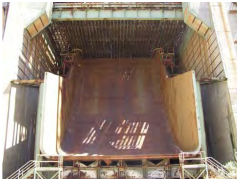
Photo 4.55. Coca IV Test Stand, flame deflector, camera facing east. (Source: Archaeological Consultants, Inc., 2007.)
