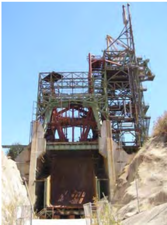
Photo 4.54. Coca IV Test Stand, east elevation. (Source: Archaeological Consultants, Inc., 2007.)
