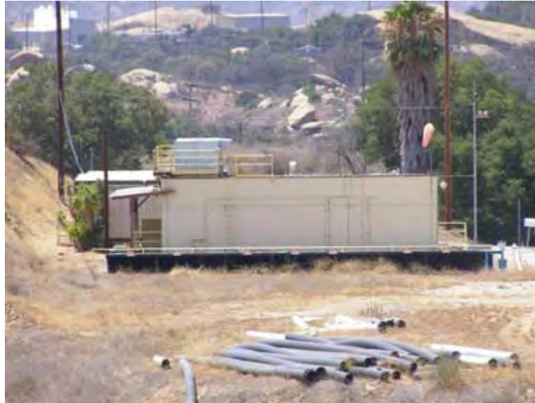
Photo 4.16. Alfa Control House, east elevation, which faces test stands. (Source: Archaeological Consultants, Inc., 2007.)
