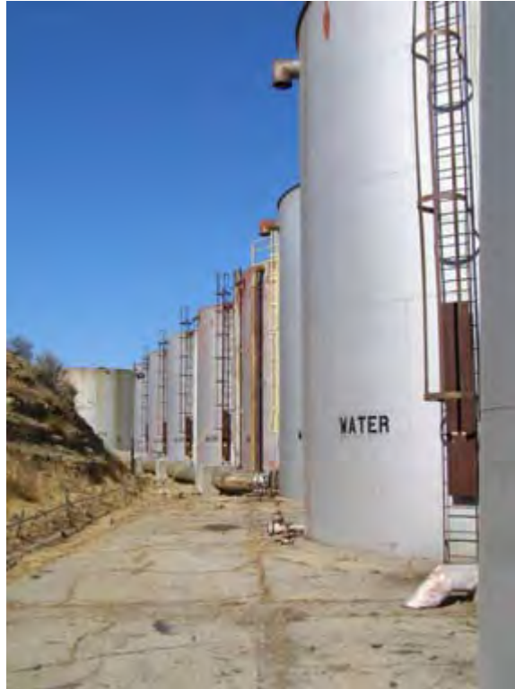
Photo 4.68. Water Tanks along Skyline Drive, camera facing west. (Source: Archaeological Consultants, Inc., 2007.)
