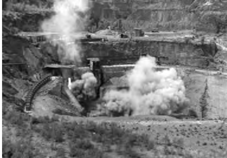
Photo 3.8. Acceptance testing of V-2 engines at an adapted quarry near Lehesten, south of Nordhausen (Mittelwerk) on the Thuringian-Bavarian border, 1945. (Source: Boeing, Rocketdyne Historic Photograph Collection, SSFL.)
