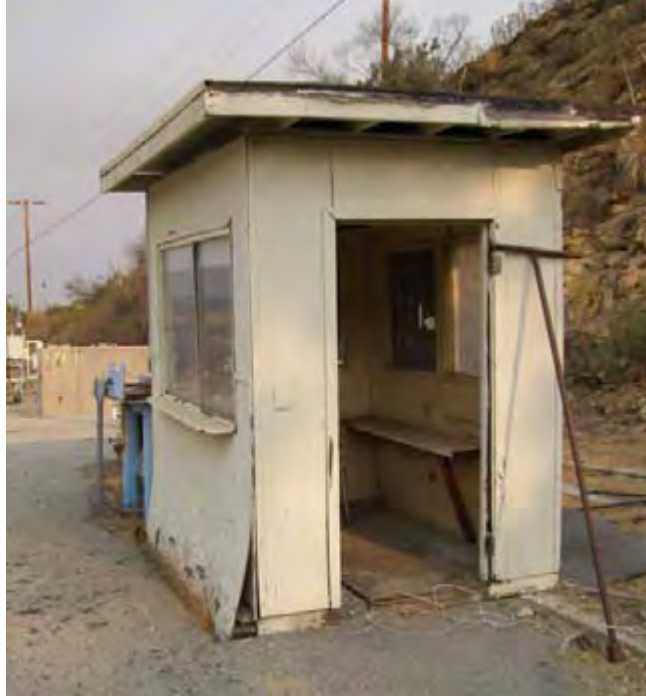
Photo 4.4. Alfa Standtalker Shack, camera facing northwest. (Source: Archaeological Consultants, Inc., 2007.)
