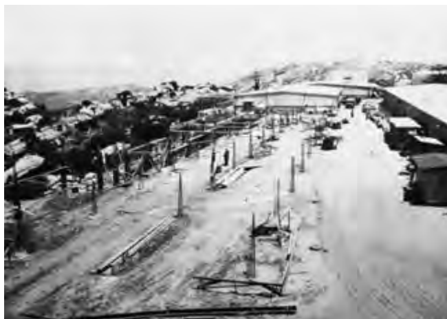
Photo 3.17. Service Area at the entrance to AFP 57 (NASA Area II), under construction, ca. 1955. (Source: Boeing, Rocketdyne Historic Photograph Collection, SSFL.)
