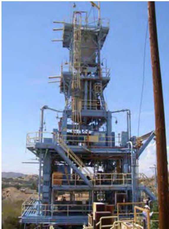
Photo 4.11. Alfa III Test Stand, east elevation. (Source: Archaeological Consultants, Inc., 2007.)
