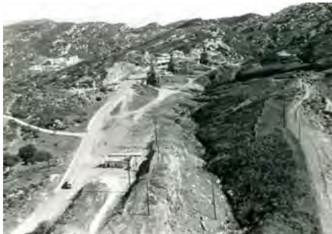
Photo 3.16. Alfa site at AFP 57 (NASA Area II), 27 January 1964. View toward the spillway ravine, underground blockhouse (center left), test stand cluster (background center), and substation on Waterwell Ridge (background left). (Source: History of the Air Force Plant Representative Office North American Aviation Rocketdyne Division Canoga Park 1 July – 31 December 1967. )
