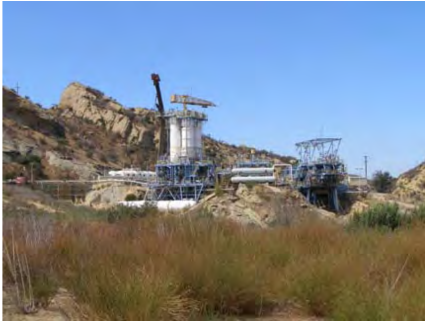
Photo 4.20. Bravo Test Area, camera facing west. (Source: Archaeological Consultants, Inc., 2007.)
