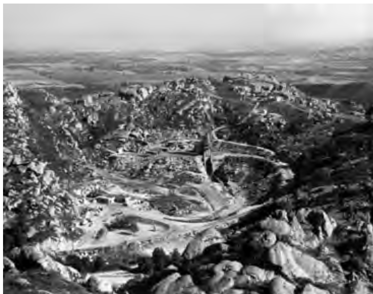
Photo 3.6. Aerial view of the Bowl Area at Santa Susana (Boeing Area I), as first completed in early 1950. Preparation stand, VTS I, blockhouse (foreground left), and two water tanks (background right of VTS I). (Source: Boeing, Rocketdyne Historic Photograph Collection, SSFL.)
