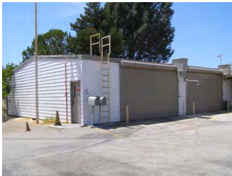
Photo 4.5. Alfa Pre-Test Building, camera facing north. (Source: Archaeological Consultants, Inc., 2007.)
