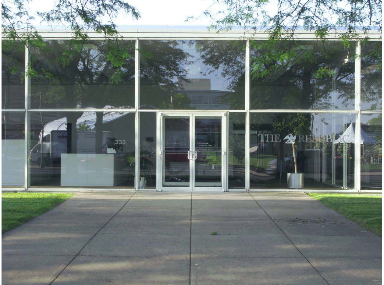
Entrance doors, north façade, looking south. Louis Joyner, photographer, 2010
