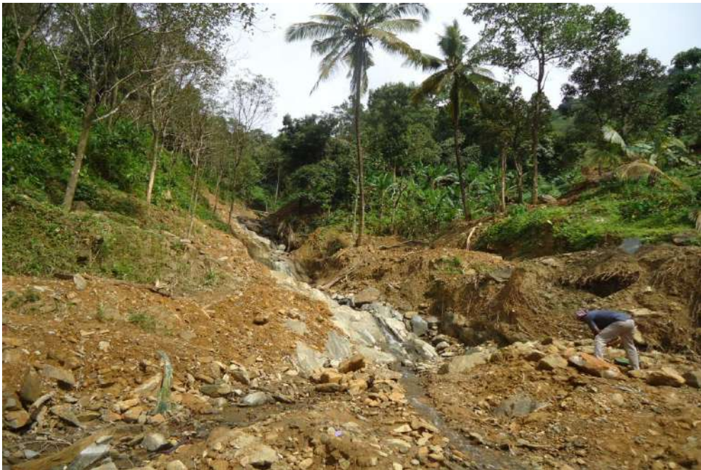
KNR/KTYR/LS-5 Mid way-Deposition occurred Santhigiri-Kelakam panchayat (cracking )
