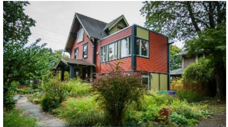
Example of an attached ADU in Portland, Oregon. Image from: https://www.portlandoregon.gov/hps/article/630137
