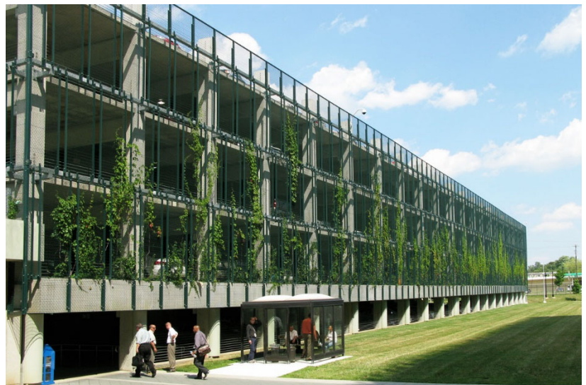
Example of early stages of a green wall parking garage screen at the Census Bureau Headquarters in Suitland, Maryland. Image from: Greenscreen http://greenscreen.com/dew/?galleries=custom
