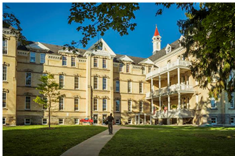
The main building, post redevelopment. Source: www.thevillagetc.com
