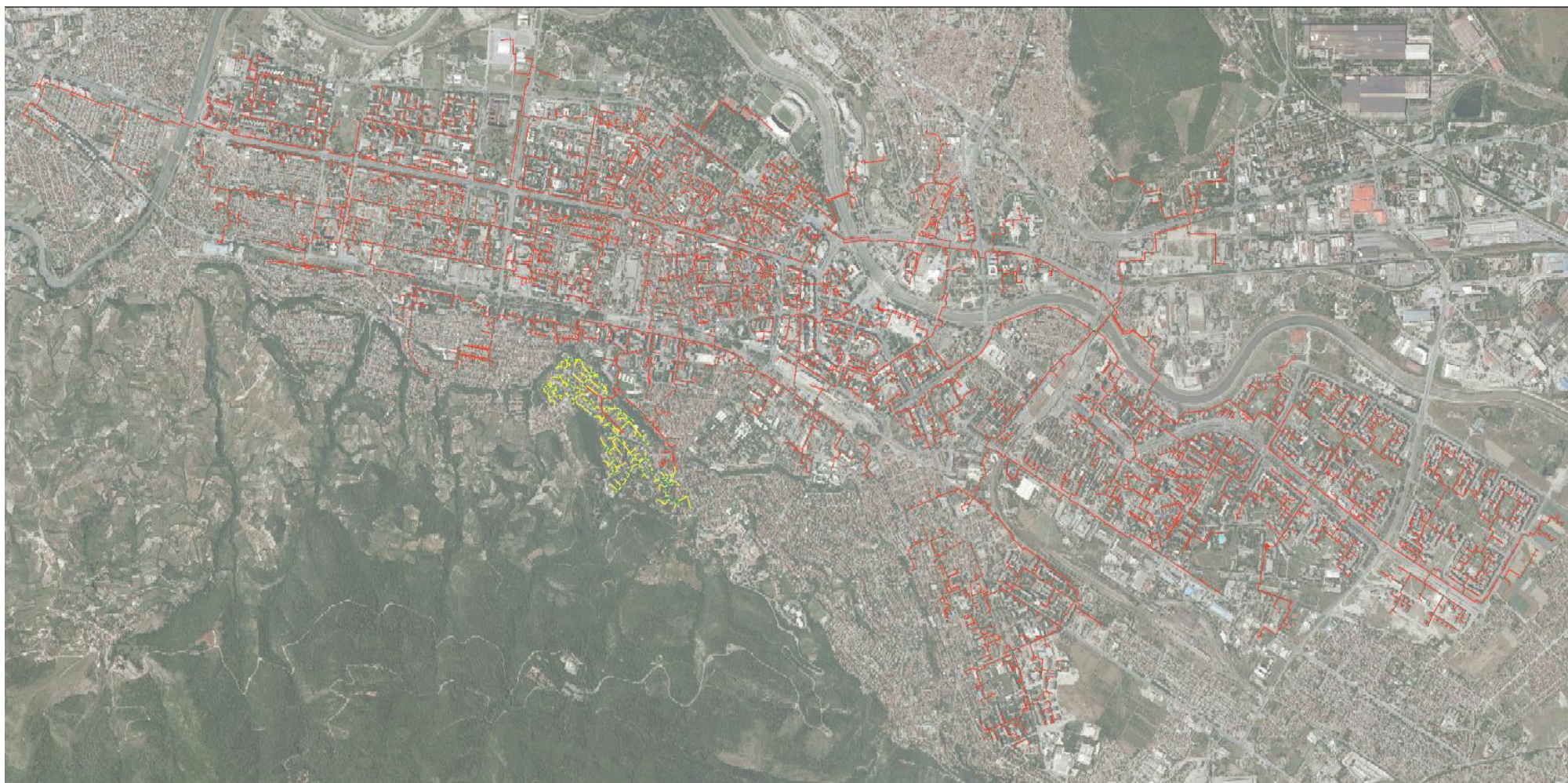
District Heating System operated by Distribucija na Toplina BE DOOEL Skopje
