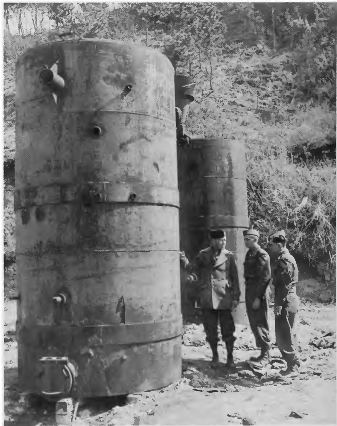
Figure 23. Rusty tanks for the hydrogen generating plant is all that remains of this former balloon launch site. Only Otsu had its own gas facilities. (U.S. Army photograph, SC 284185)
