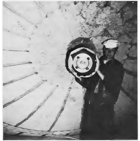
Figure 7. Imperial Japanese Navy’s balloon development consisted of a rubberized-silk envelope. Due to the weight, its payload was much less than the paper balloon developed by the army. (U.S. Air Force photograph, 30770).
