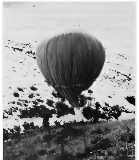
Figure 4. A faulty ballast-dropping mechanism caused this balloon to land, without dropping its bombs, near Tremonton, Utah, on 23 February 1945. Little damage was caused to the envelope.
