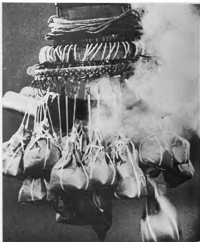
Figure 67. The bomb load and full ballast attached to a Japanese balloon gondola. Exploding blowout plug releases a sandbag shown in this movie still. The cycles continue, finally releasing the two incendiaries at left and the 33-pound, anti-personnel bomb which hangs nose down in the center. (29910 AC)
