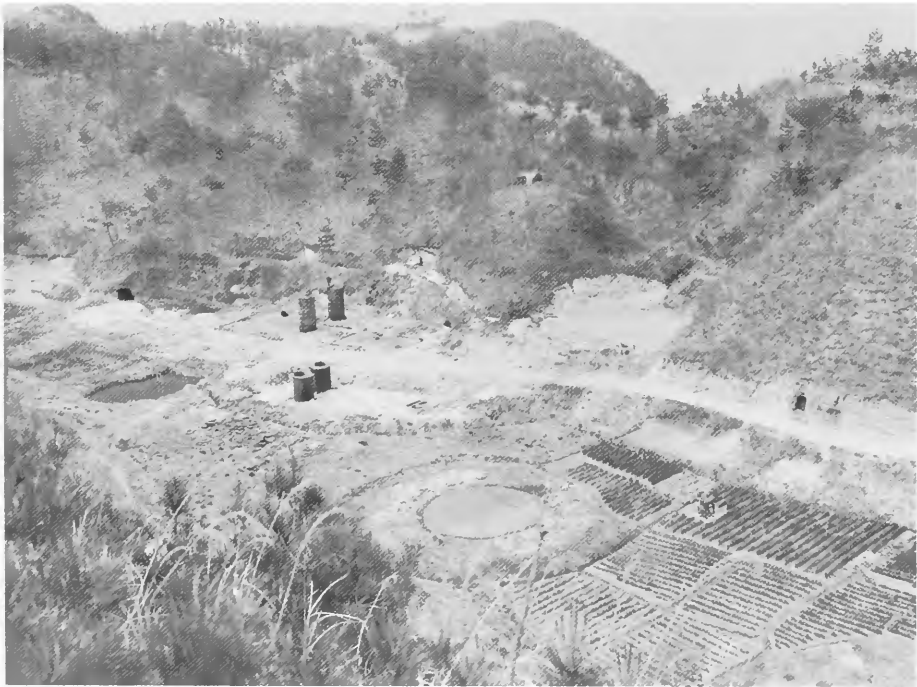
Figure 17. Balloon launching complex at Otsu after the war. Note the shelter caves in the side of the hills and the sea in the background. (U.S. Army photograph, SC 284816)
