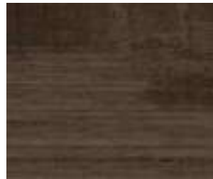
Dinding Beton expose Tanpa finishing
