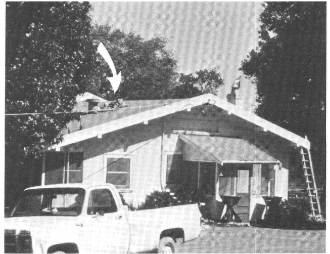
Figure 11.15. Damaged wood-frame house (built about 1914) in the San Felipe Valley. Chimney toppled (arrow) and stemwall cracks developed in perimeter foundation. View east-southeastward.
