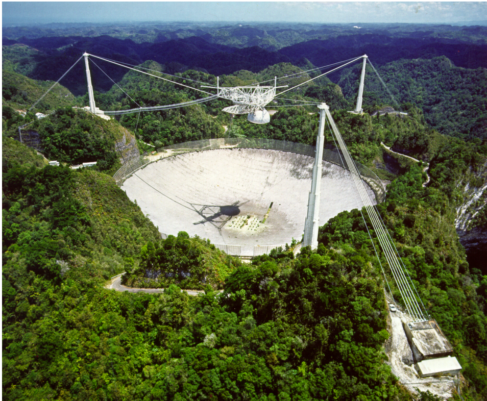
Figure 2.5 The 300 metre dish at the Arecibo Observatory in Puerto Rico. It was used by radio amateurs for EME communication in 1964, 1965 and 2010. (Photo courtesy of the NAIC – Arecibo Observatory [114], a facility of the NSF .)
