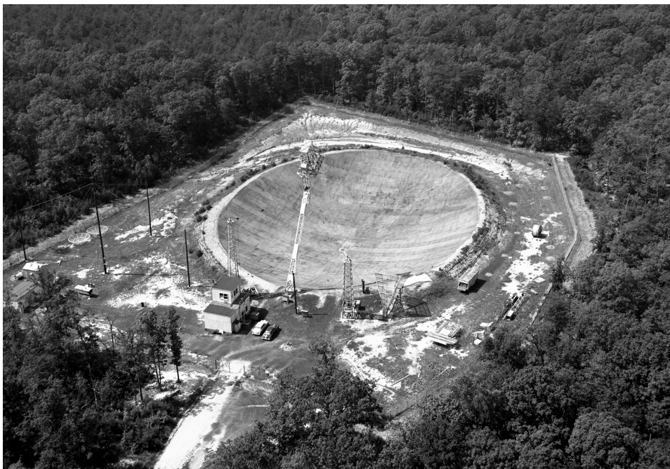
Figure 2.2 The NRL's Stump Neck site with the 67 by 80 metres elliptical parabola. The focal point is approximately 27 metres above the dish, where a horn-type feed is used. The gain and beam width were measured using the Sun as well as a 'horn gain standard', which can be seen on the ground to the right of the parabola. (Photo courtesy of the NRL [115].)
