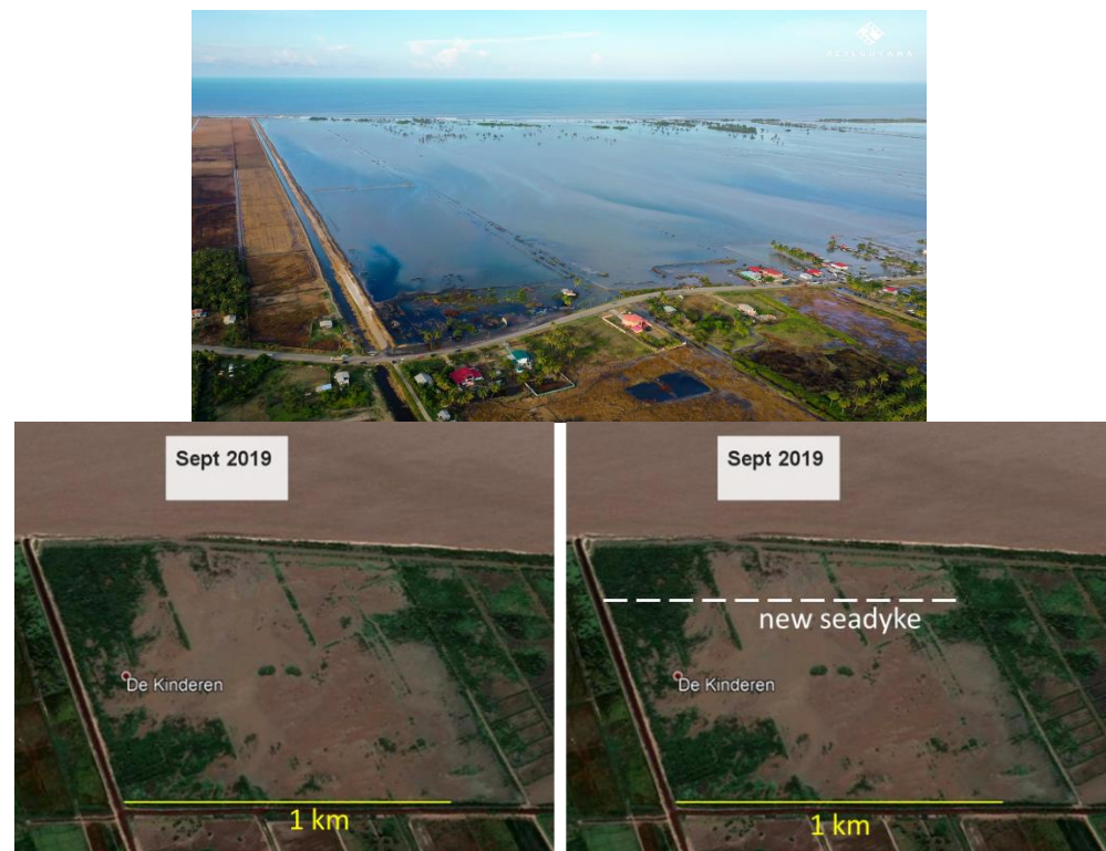
Figure 8.1 Upper panel: breaching and inundation near De Kinderen; lower left panel: keep entire inundated polder open for sediment-laden water to enter; lower right panel: erect new embankment/seawall 100 – 200 m inland from the original one.
