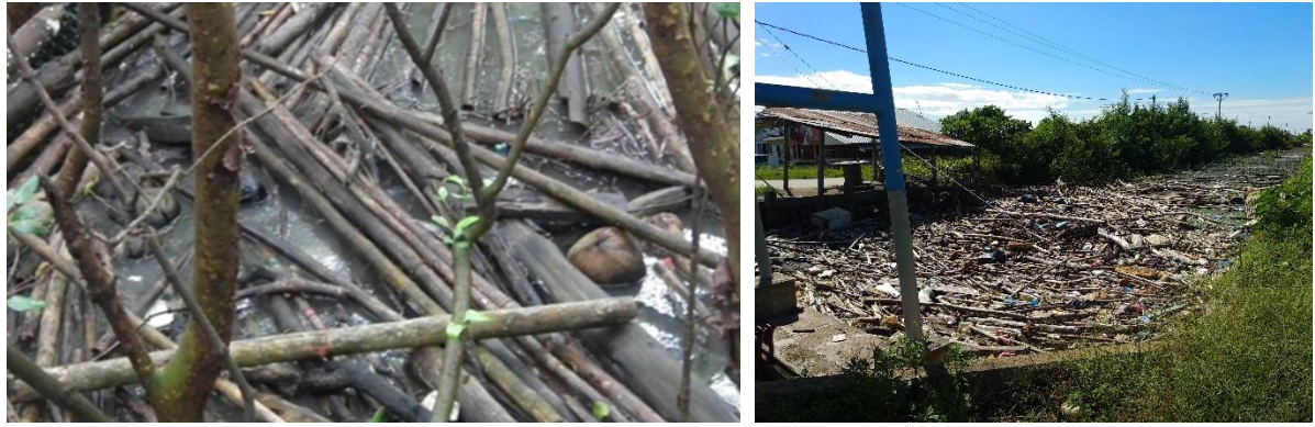
Figure 7.9 Debris from permeable structures in mangrove forest, Thailand (left panel, courtesy Cherdvong Saengsupavanich) and in a drainage channel near Weg aan Zee, Paramaribo, Suriname (right panel, courtesy Els van Lavieren)
