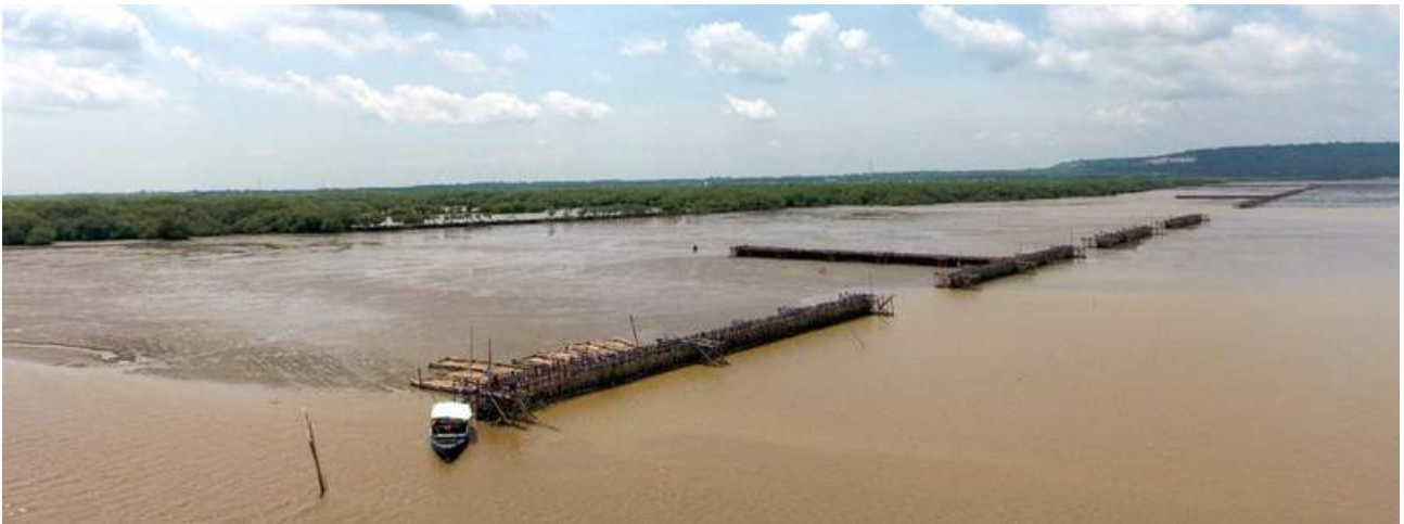
Figure 12. MudBank Motor concept to accelerate natural mudflat formation behind mudbanks and protect existing mangrove fringes
