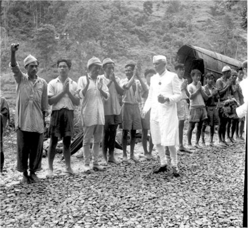
Prime Minister with workers who constructed a road for his journey to Bhutan on September 16, 1958.
