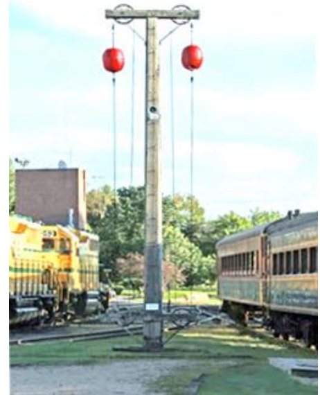
Here is a danger ahead signal at North Conway, New Hampshire. Image from archlapeer
