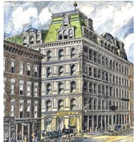
Shown is the time ball mounted on the roof of the Carlisle Building at Fourth and Walnut Streets. Image from Phorio (Public Library of Cincinnati and Hamilton County. Genealogy & Local History Department). Illustrated News – Great Exposition Number, August 21, 1886, page 17.
