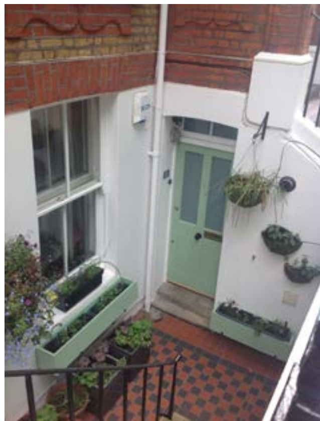
Original basement door and traditional cast iron door knob
