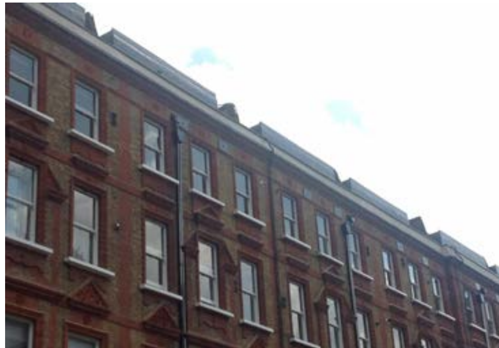
Unsympathetic roof additions
