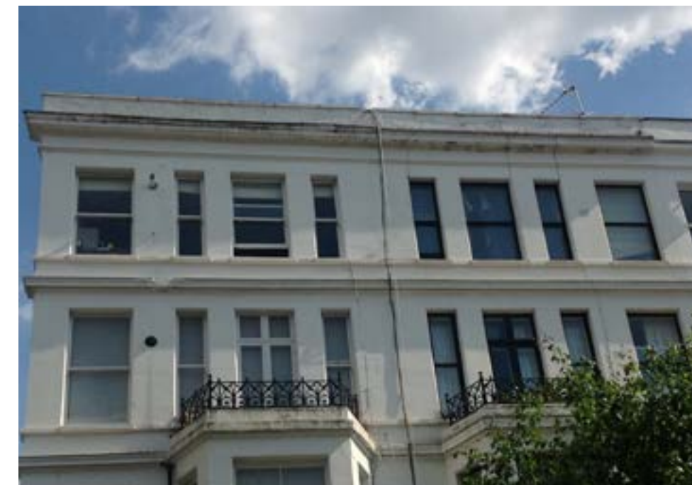
Plain parapet and cornice concealing roof, Longridge Road
