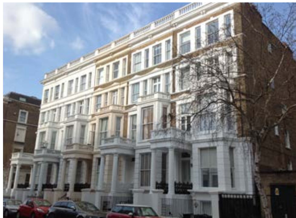
Nos. 2-10 (even) Nevern Road
