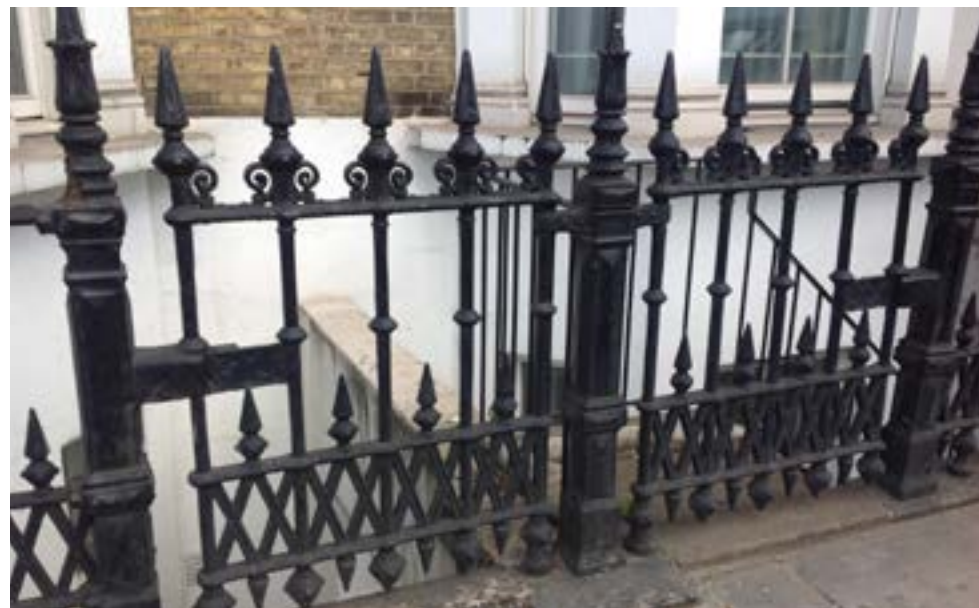
Iron railings, Warwick Road
