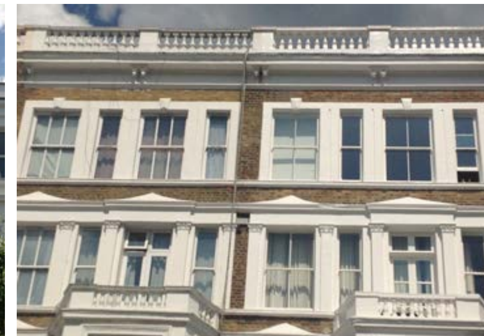
Classically inspired parapet with balustrade and bracketed cornice, Nevern Road
