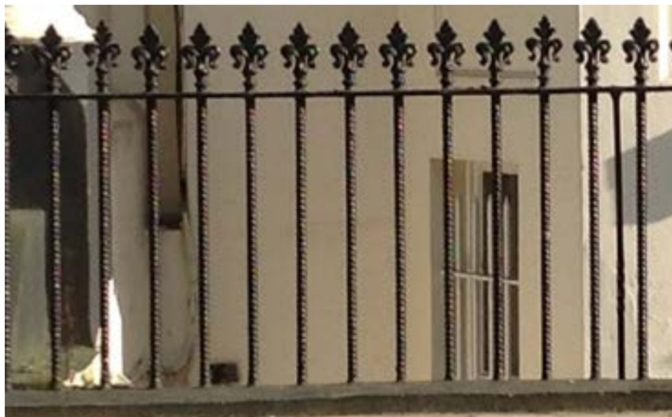
Iron railings with twisted posts, Nevern Place
