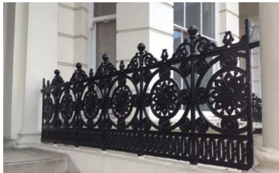
Iron panel to entrance, Nevern Place
