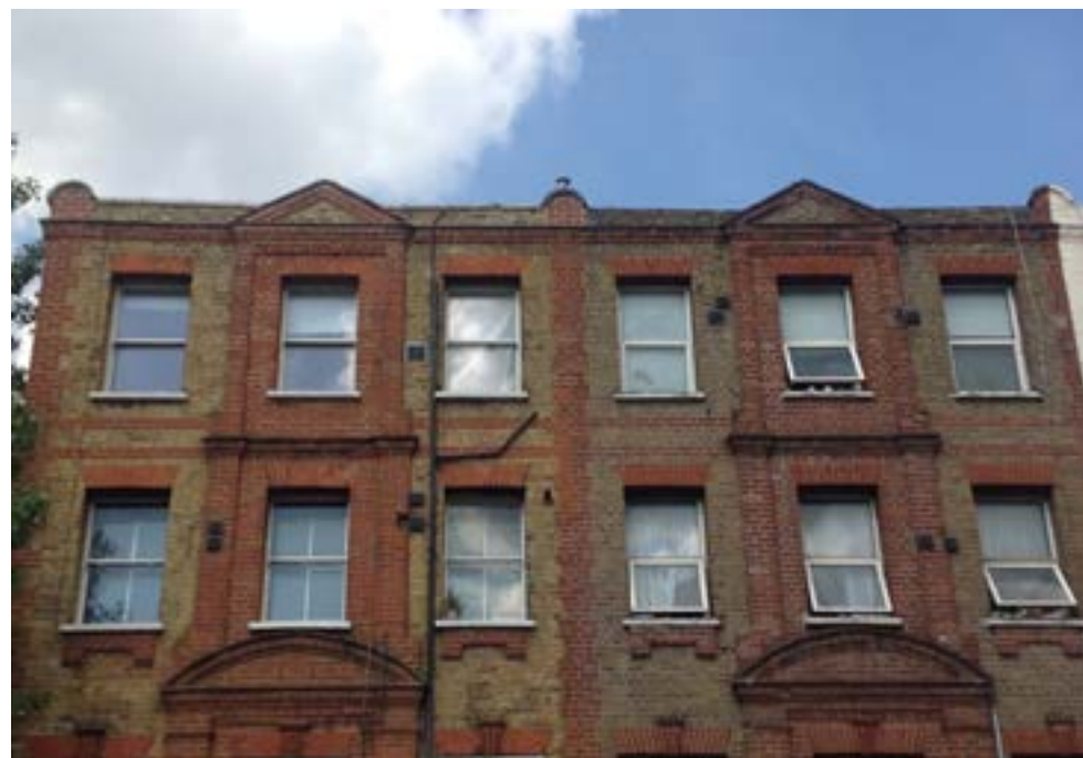
Stock brick parapet with red brick pediments and detailing, Warwick Road
