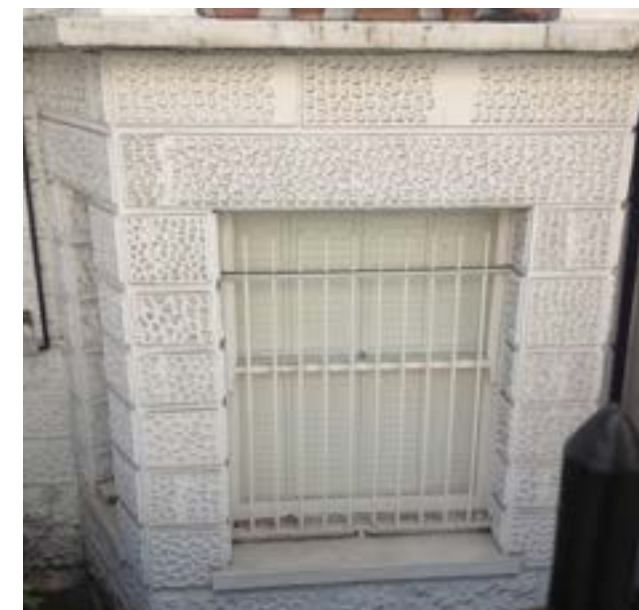
Rusticated basement bay window
