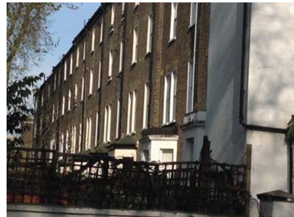
Rears of nos. 2-24 (even) Nevern Place
