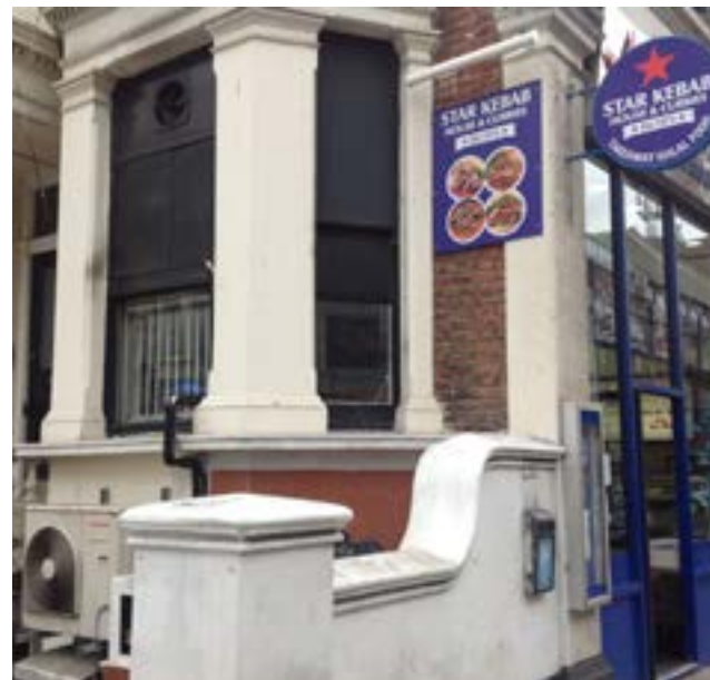
Signage, blocked window and extraction unit
