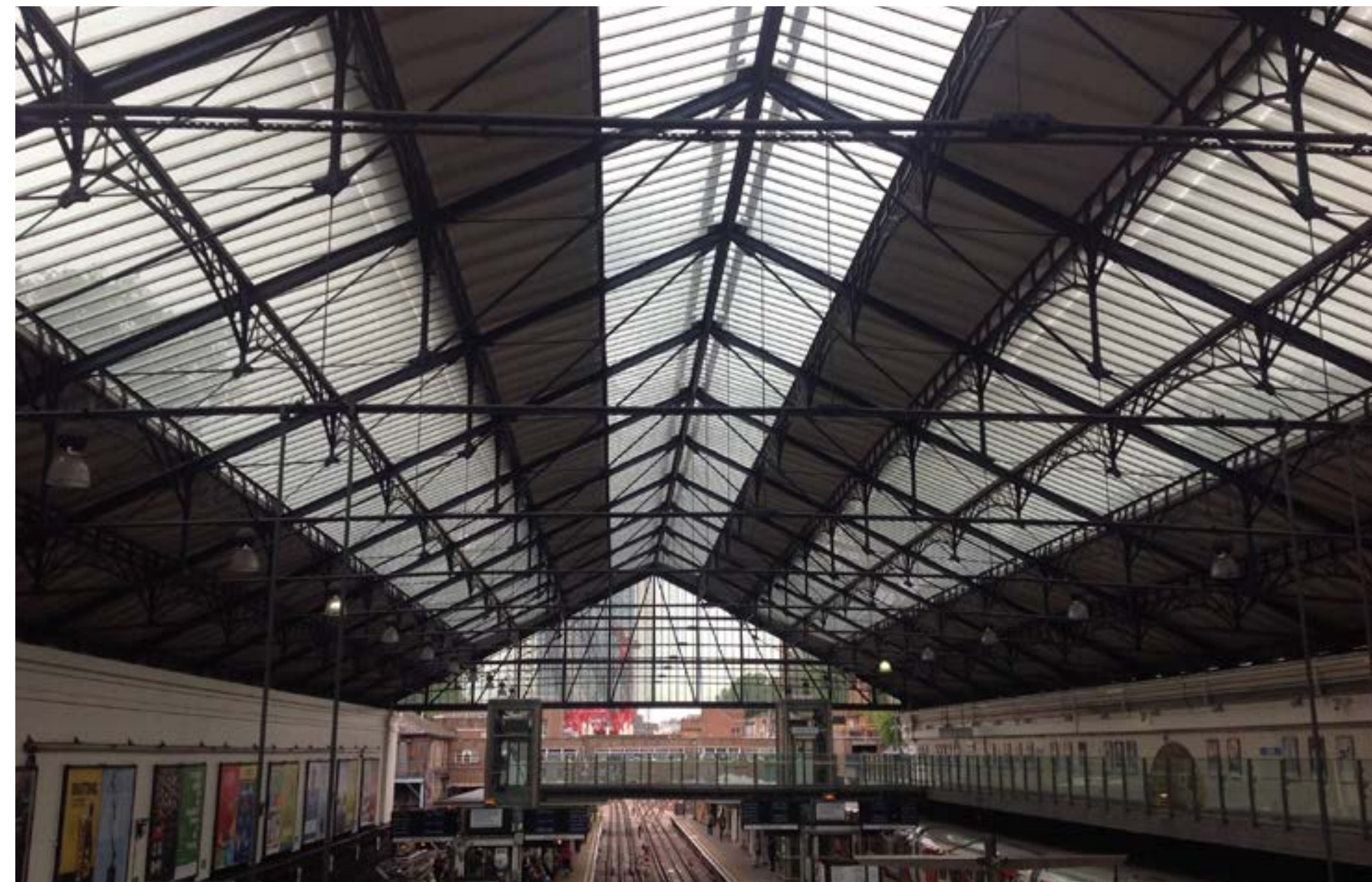
Earl's Court Station roof
