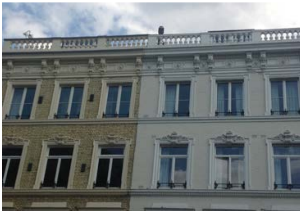
Classically inspired parapet with balustrade and bracketed cornice, Trebovir Road
