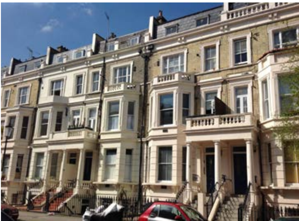
Nos. 6-12 (even) Longridge Road
