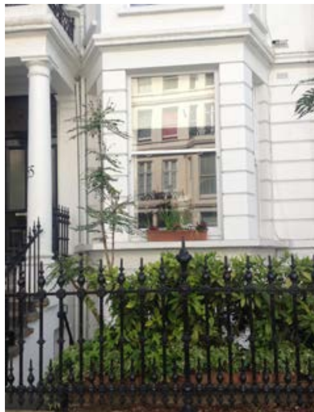
Original cast iron railings, Longridge Road
