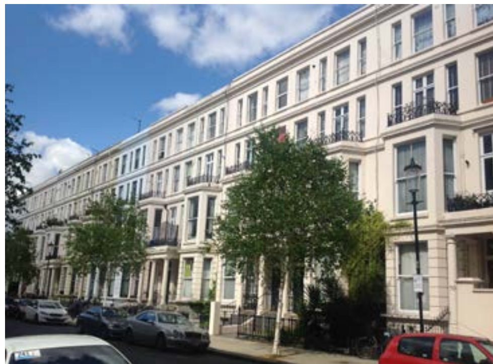
Nos. 50-70 (even) Longridge Road
