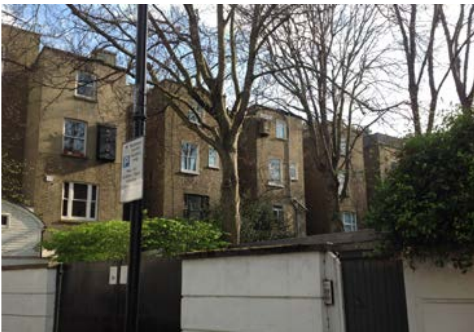
Rears of nos. 26-34 (even) Nevern Place
