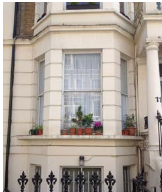
Plain timber framed, single glazed sash windows in Italianate channelled bays
