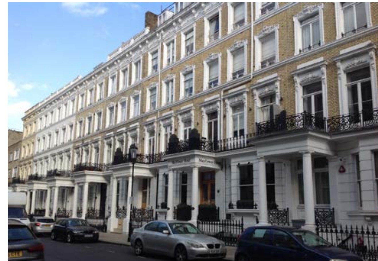
Nos. 16-32 (even) Trebovir Road
