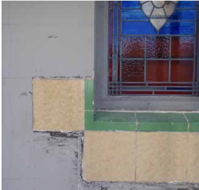
Original faience beneath modern paint finishes and coloured decorative leaded windows to The King's Head public house
