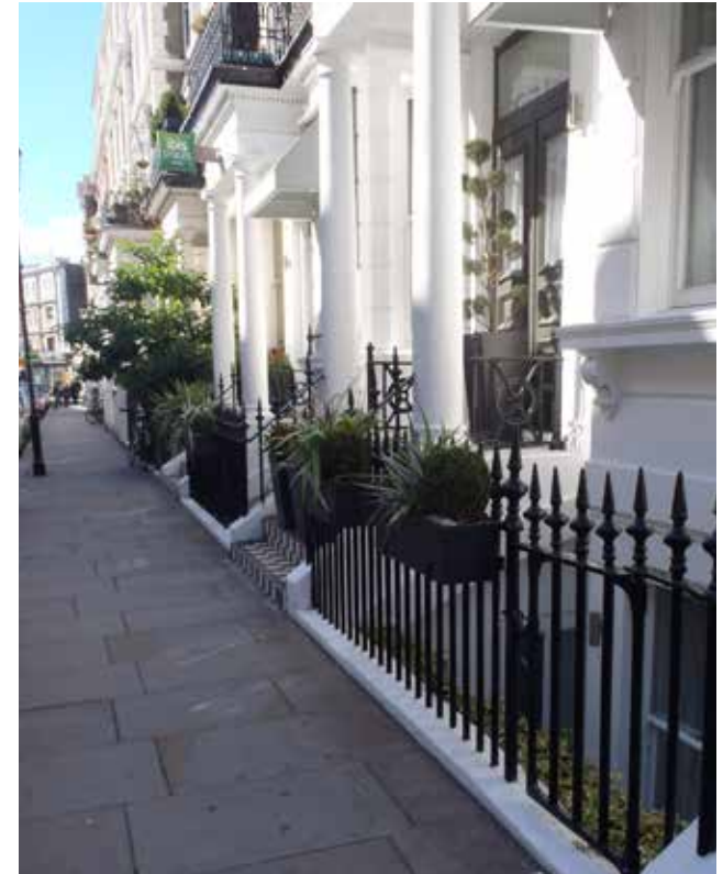
Planting behind railings in Hogarth Place
