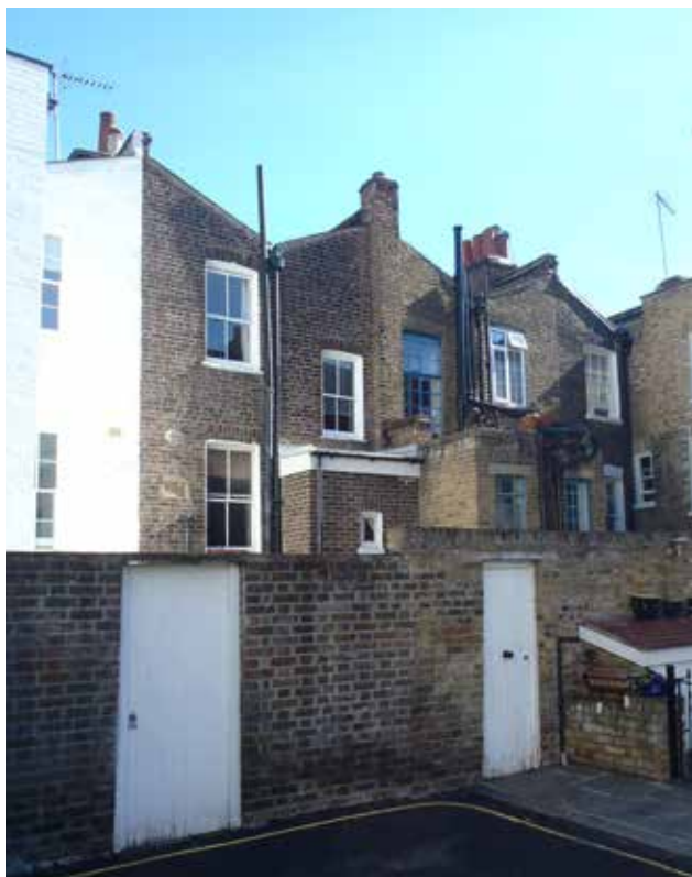
Rear elevations of Wallgrave Road from Child's Street
