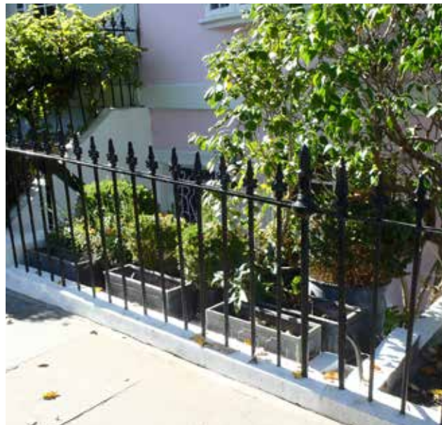
Cast iron railings
