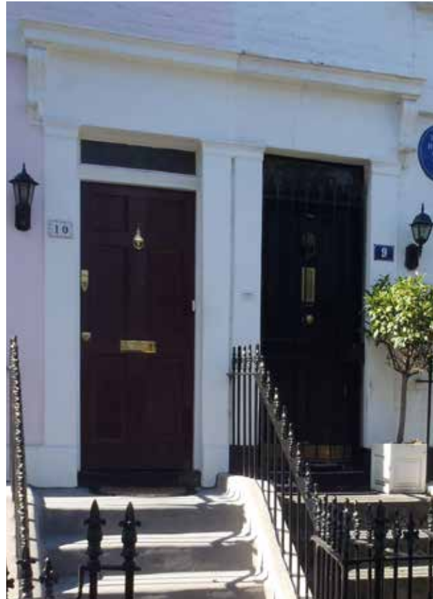
Six panelled doors, Wallgrave Road
