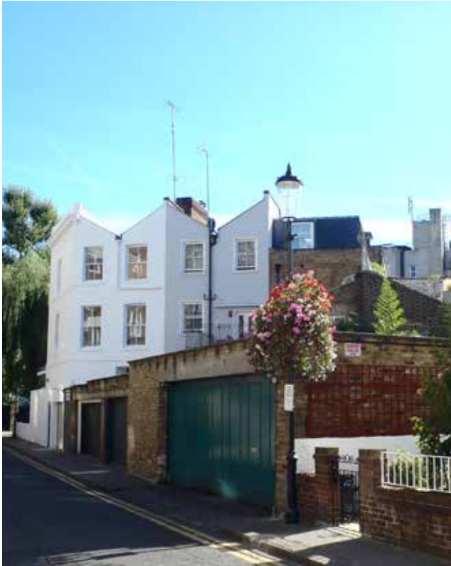
London roofs to rear of nos. 73-77 (odd) Kenway Road
