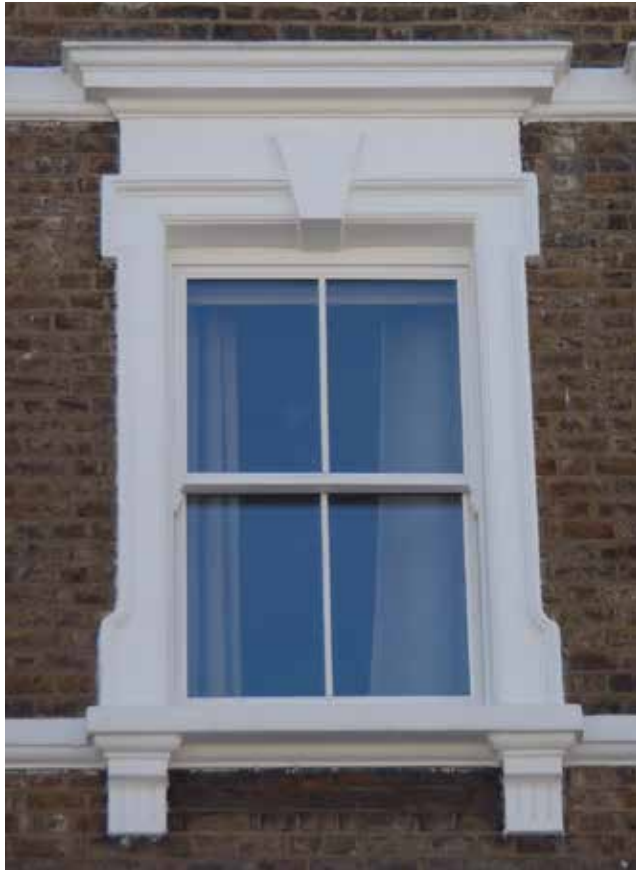
Traditional sash window with decorative architrave surround, Hogarth Road
