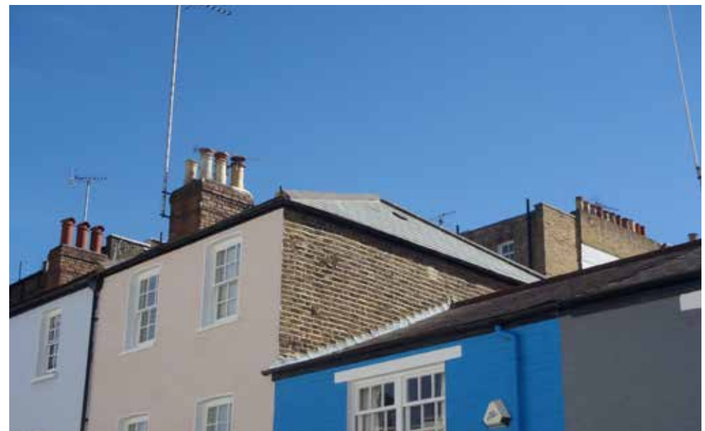
Hipped roof, Kenway Road
