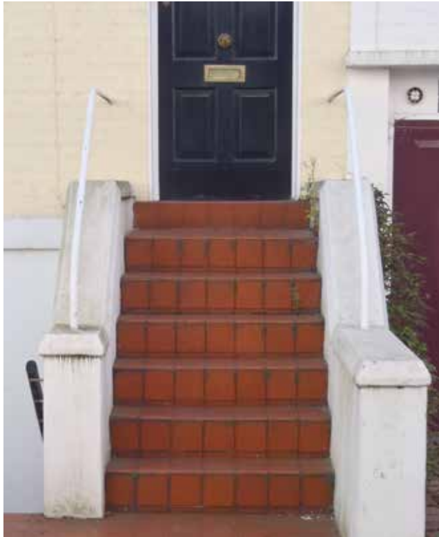
Replacement coverings to entrance steps
