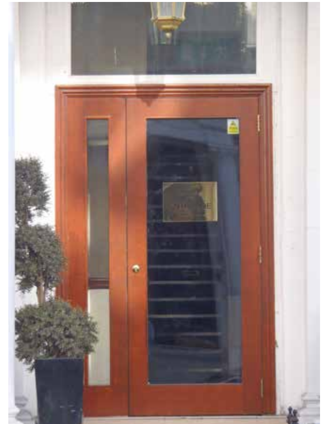
Modern replacement doors
