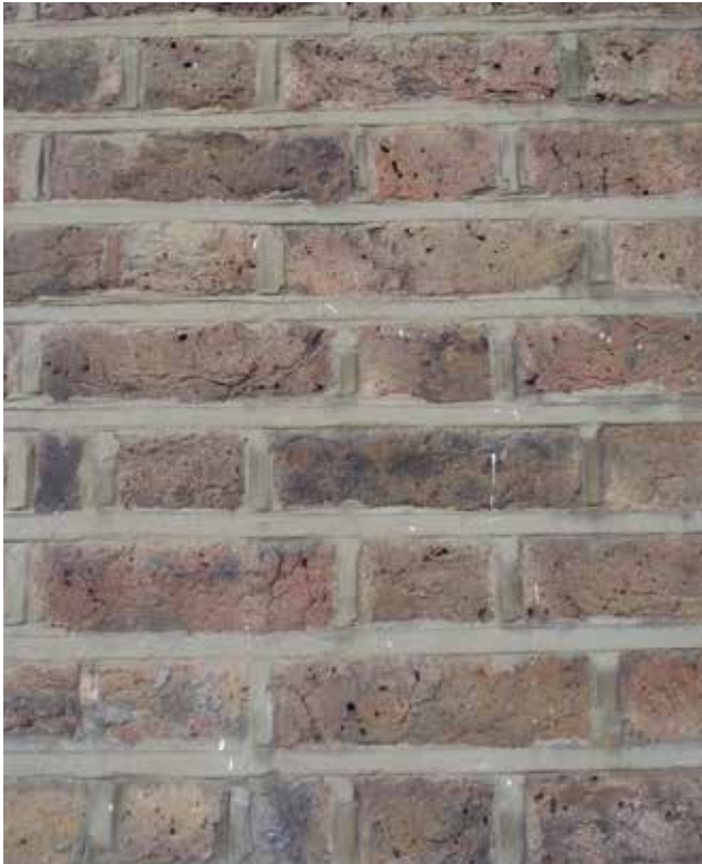
Weather struck cement pointing
