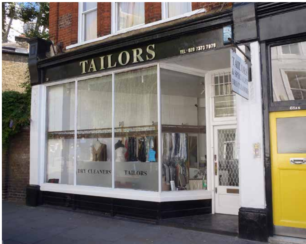
Original Victorian shopfront to no. 70 Kenway Road
