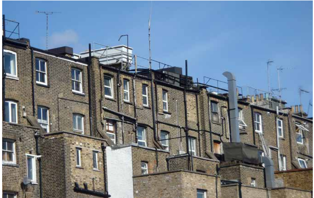
External clutter with the addition of pipework, railings, tanks and flues
