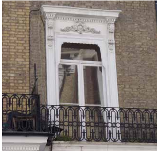
French doors set within decorative architrave surround, Hogarth Road
