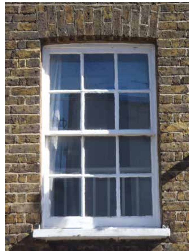
Six-over-six sash windows with cambered brick head, Wallgrave Road
