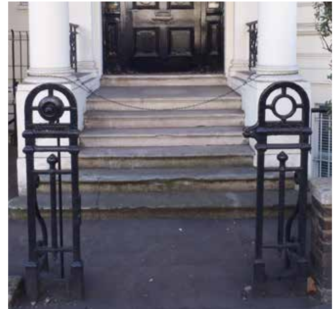
Decorative cast iron gate posts, Cromwell Road
