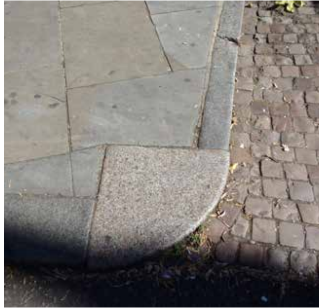
York stone paving slabs, granite kerb stones and stone setts
