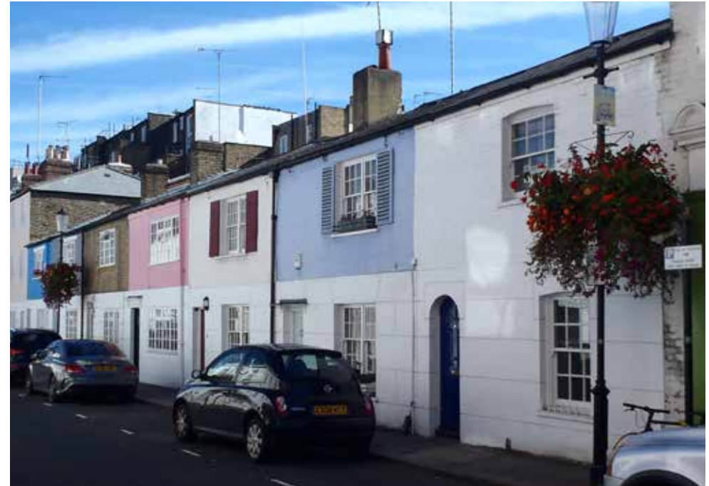
Nos. 18-30 (even) Kenway Road
