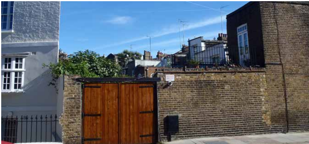
Gap between no. 35 Kenway Road and no. 18 Wallgrave Road
