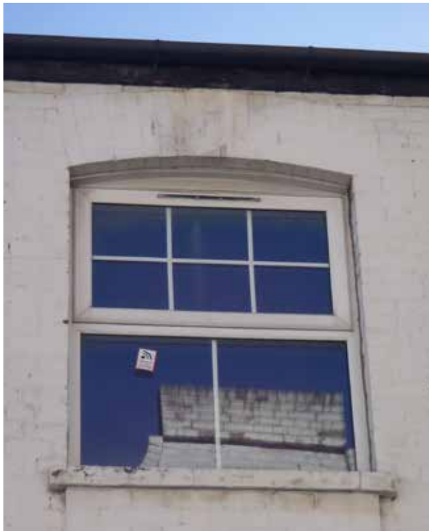
uPVC replacement windows
