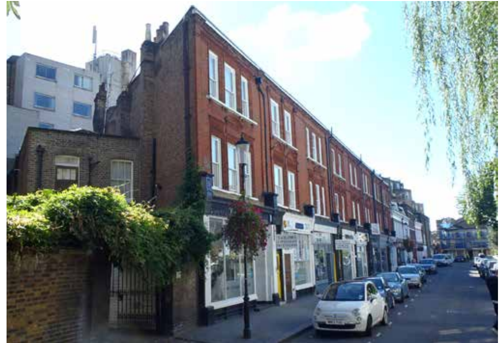
Nos. 56-70 (even) Kenway Road
