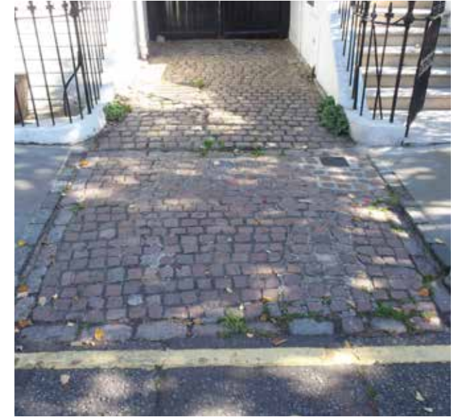
Stone setts to covered carriage way, Wallgrave Road
