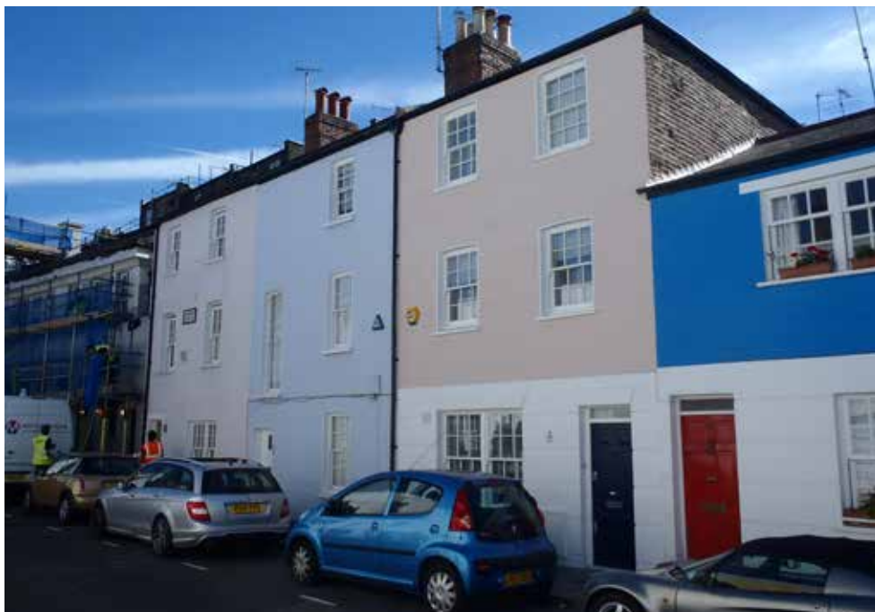
Nos. 32-36 (even) Kenway Road
