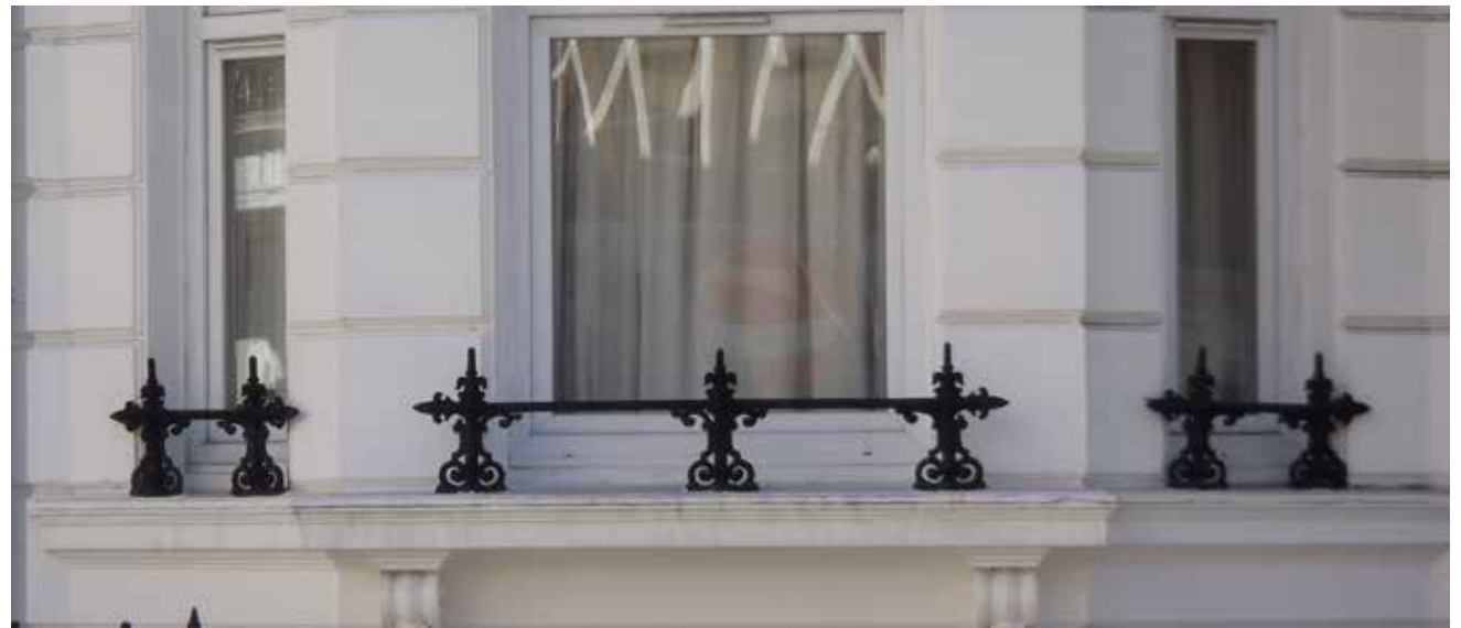
Pot guards to houses within Knaresborough Place
