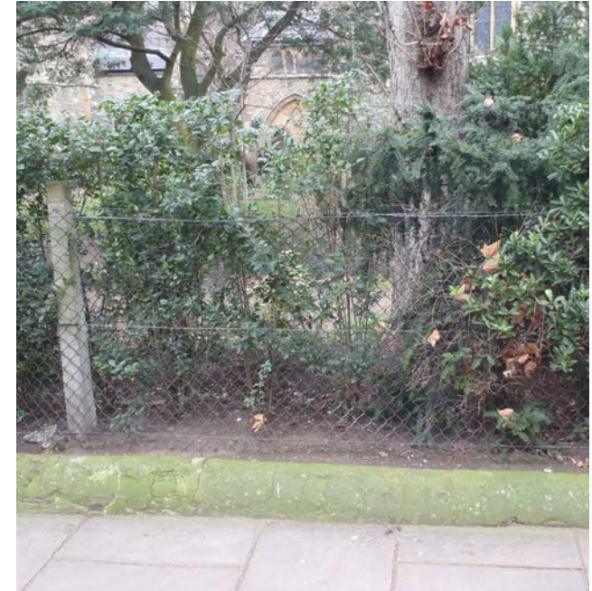
Wire fence to St. Jude's Church
