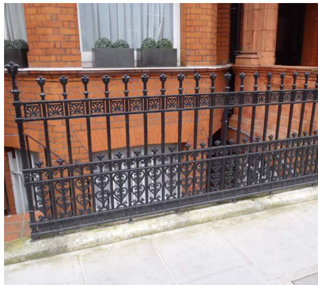
Original railings, Bina Gardens
