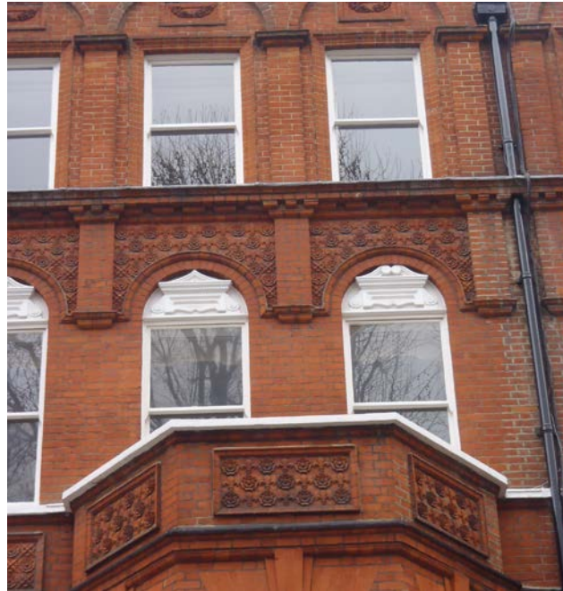
One over one wooden sash windows, Barkston Gardens
