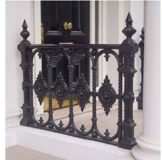
Railings to Portico 31 Collingham Road
