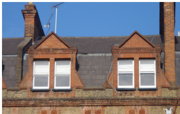
Rear mansard and dormers to Courtfield Road
