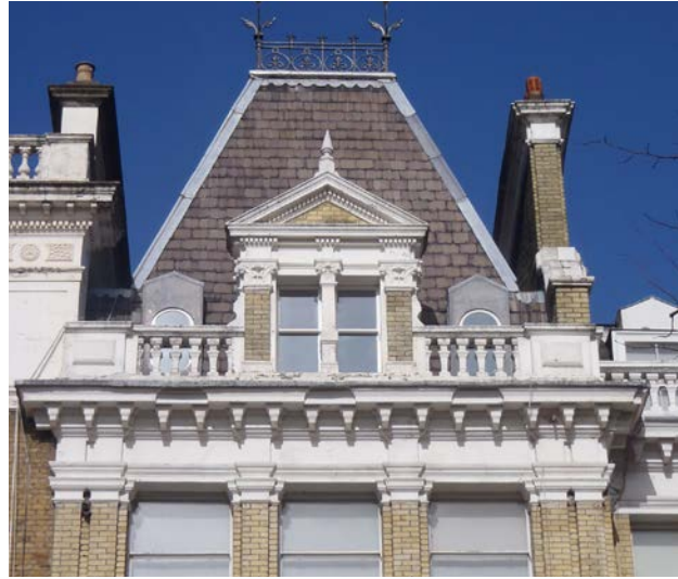
Gault brick and ornate stucco dressings
