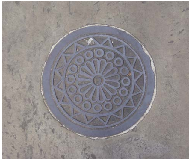
Coal hole cover, Bolton Gardens
