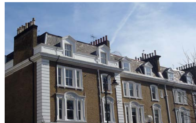
Mansard roofs, 14-15 Boltons Gardens
