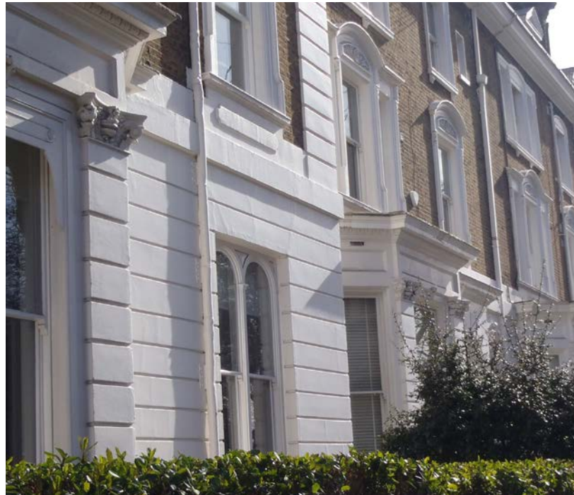
Rusticated stucco and London stock brick
