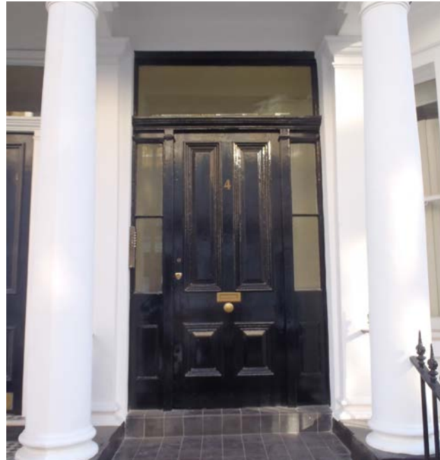
Four panelled door Courtfield Gardens
