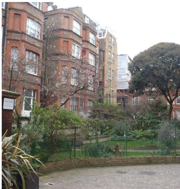
14-30 Bina Gardens (rear)
