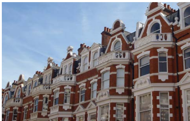
Roofs along Boltons Gardens
