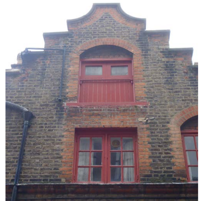
Pitching door and side hung casement window, Colbeck Mews
