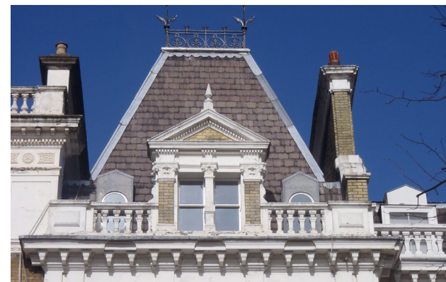
Ornate dormer and steeply pitched roof, 12 Wetherby Gardens
