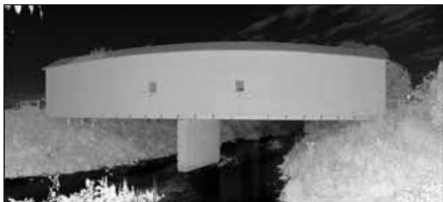
Figure 30. Scalar image of the outside of the Zumbrota Bridge created from a single exterior scan processed with Faro Scene software.
