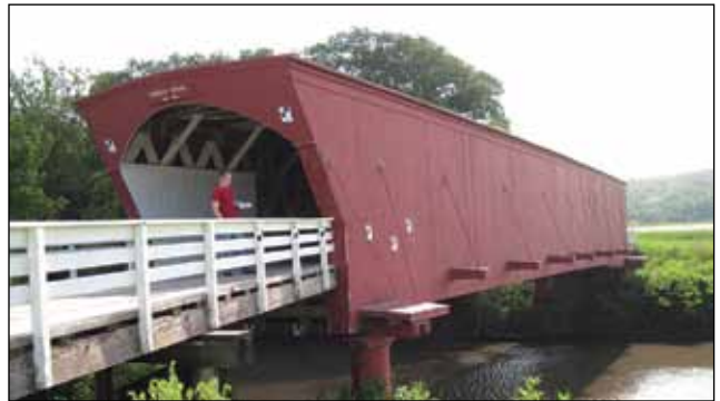
Figure 5. Hogback Bridge, Madison County, Iowa (2010).
