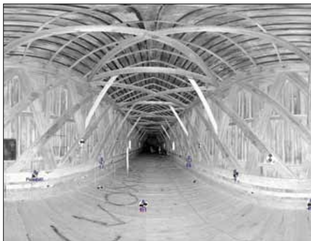
Figure 31. Scalar image of the inside of the Zumbrota Bridge created from a single interior scan processed with Faro Scene software.
