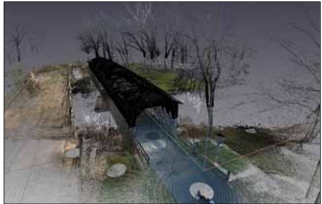
Figure 10. Point cloud image of the Cedarburg Bridge (SightLine, LLC).
