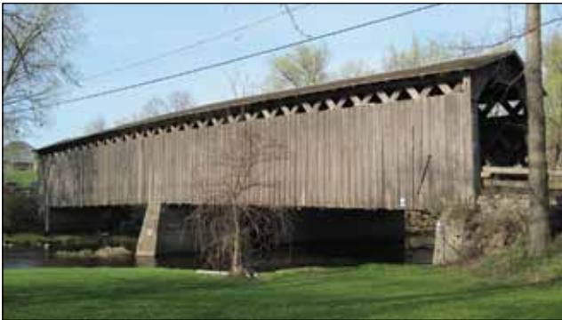
Figure 2. Recent (2010) photograph of the Cedarburg Covered Bridge.
