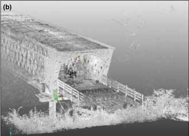
Figure 25. Point cloud images of the Roseman Bridge (NRR).
