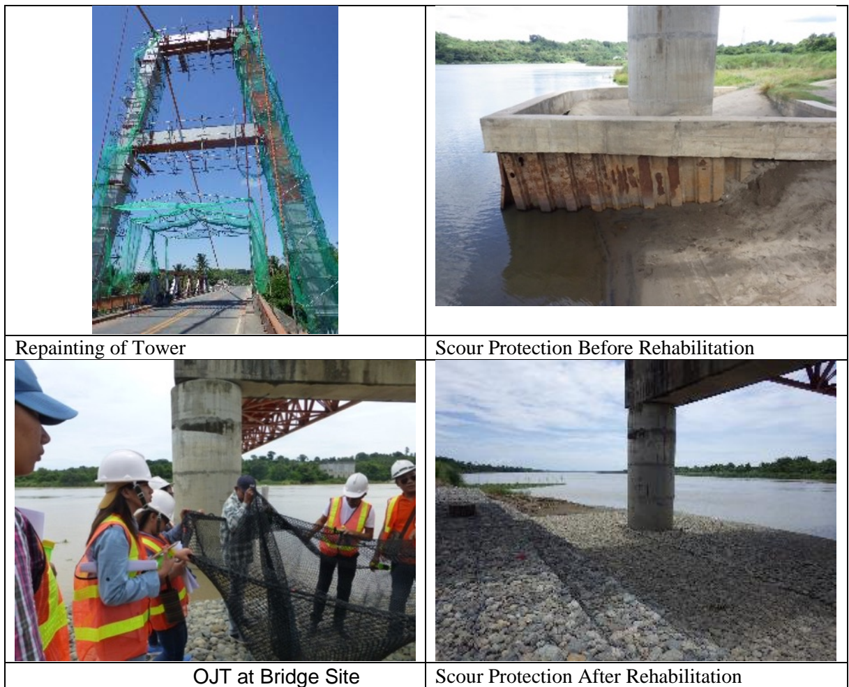
Figure 1.3.3.4-3 Activities in Stage-2
