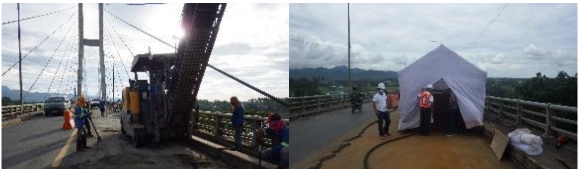
Figure 1.3.3.4-12 Removal of Existing Asphalt by Scarifier
