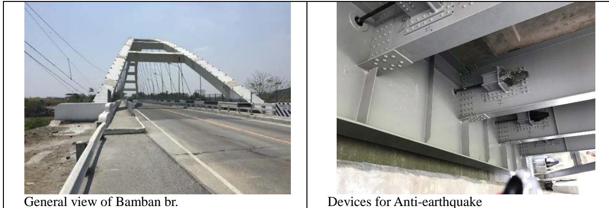
Figure 1.3.3.4-7 Bamban Bridge and Devices for Anti-earthquake
