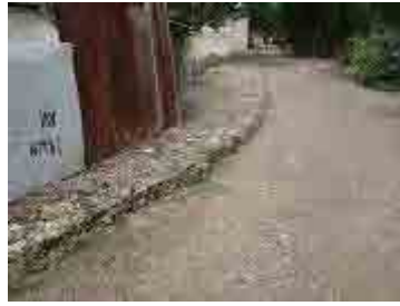
Former dike (1.9km on left bank)
