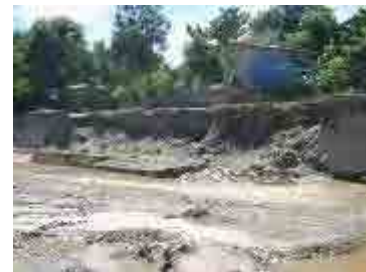
Collapsed Revetment
