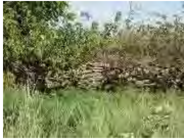
Former masonry revetment (0.7km on left bank)
