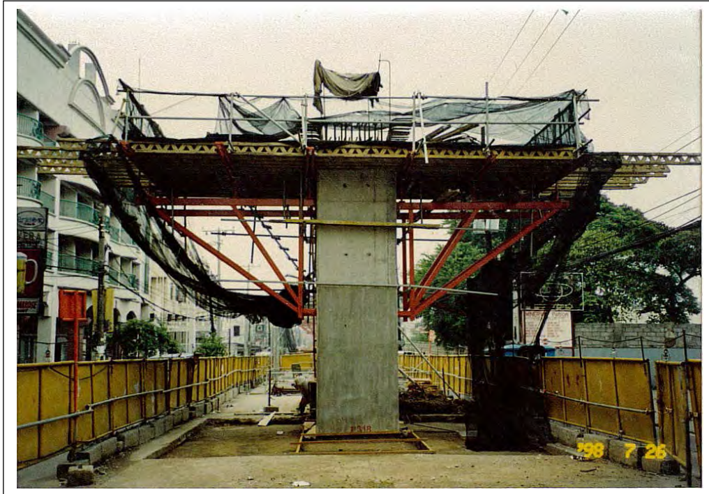
Photo 5.1-2 Pier Column Construction – LRT Line 2
