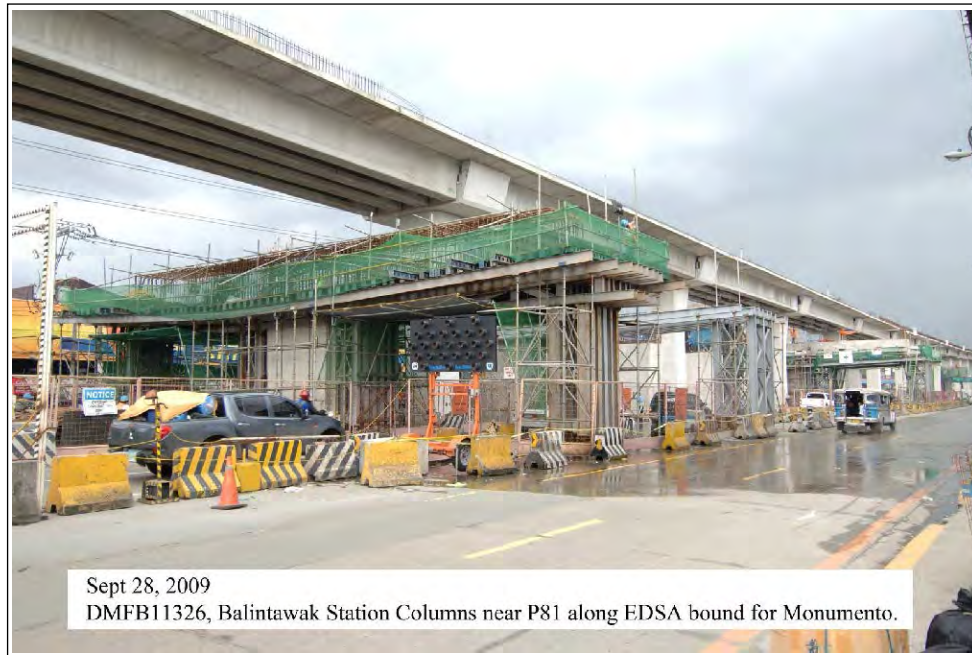
Photo 5.1-6 Station Cantilever Pier Construction – LRT Line 1 NEP
