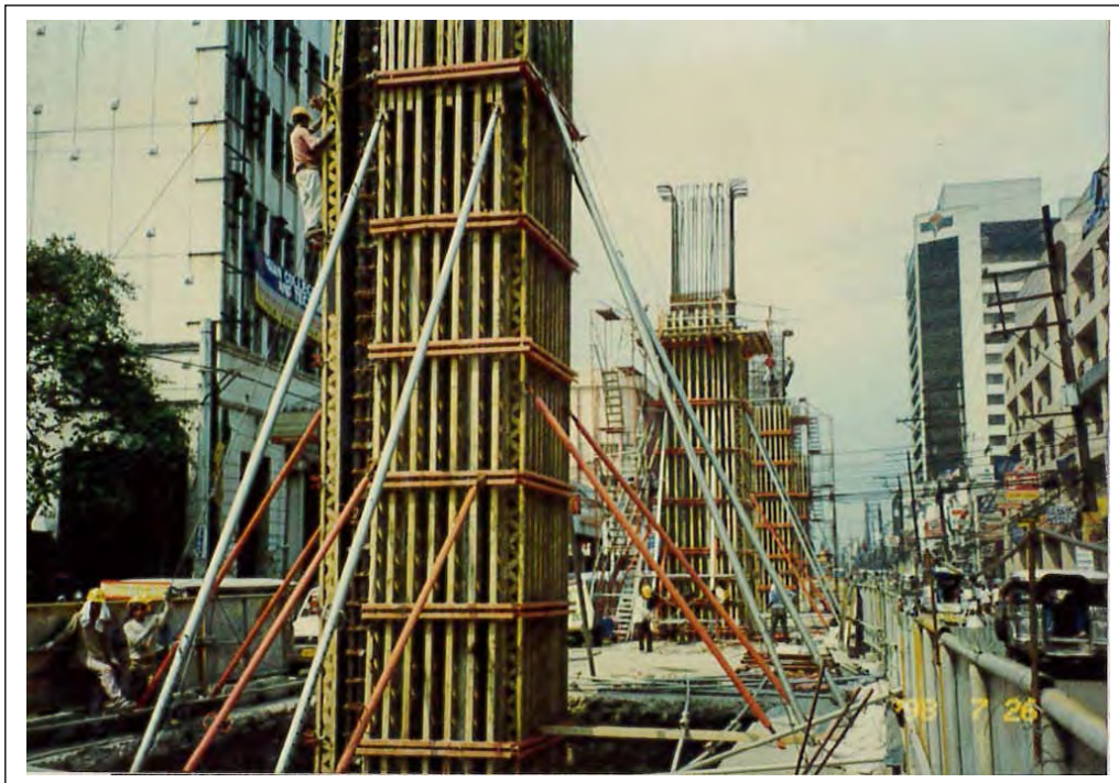
Photo 5.1-1 Pier Column Construction – LRT Line 2
