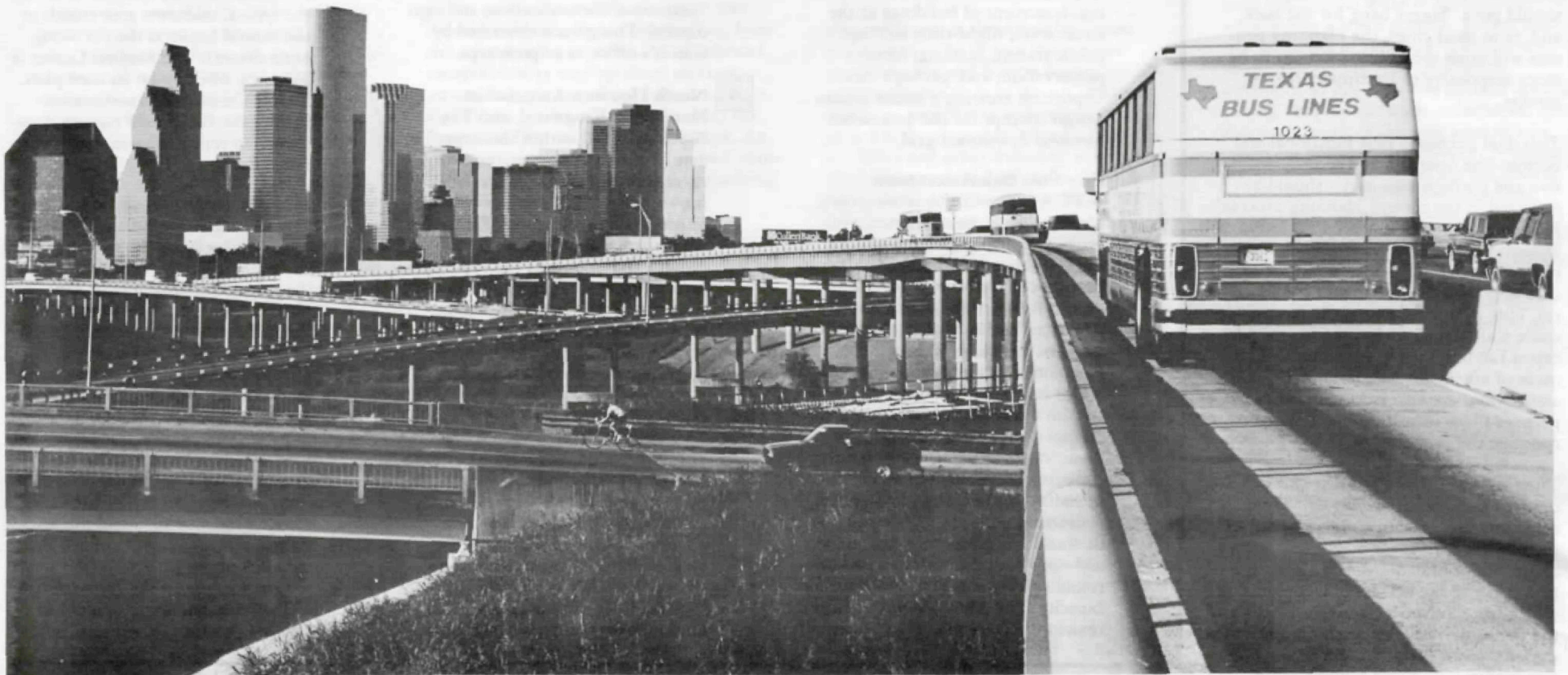
The median bus/van lane in the North Freeway (I-45) carried as many passengers as automobiles in three adjacent freeway lanes in peak periods (Photos by Paul Hester)
