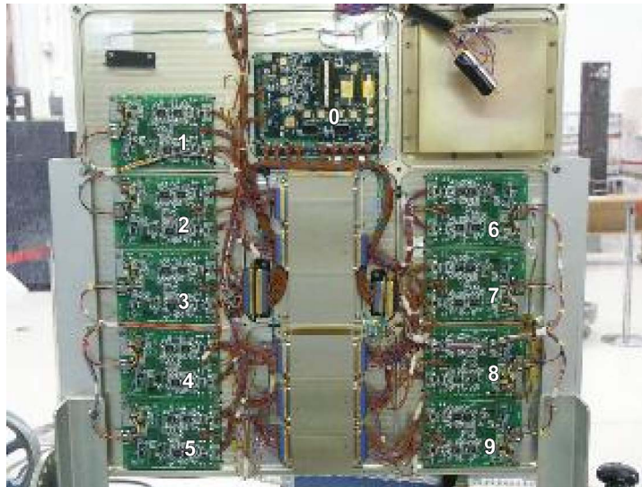
Figure 20. Photograph of the DAC (1-9) boards and main microprocessor board (0) that perform the FTSCE electrical measurements. The metal box in the upper right is the power control unit (PCU). The metal boxes in the center route wires from the solar cells mounted on the opposite side and serve to maintain a Faraday cage around the measurement electronics. 18
